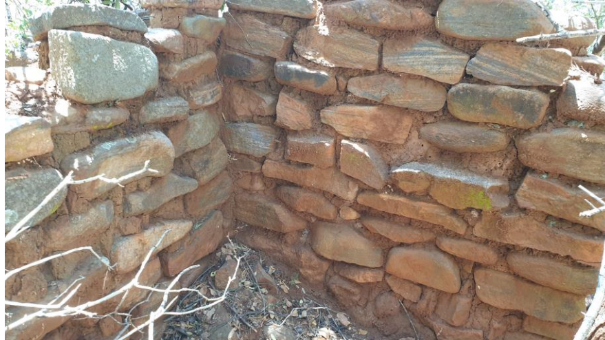
Figure 37: Detail of the inside of the stone wall indicating mud in fill between the rocks
