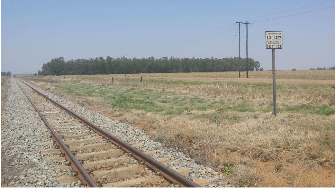
Photo 1: Road, Railway and Power line passing through the prospecting area
