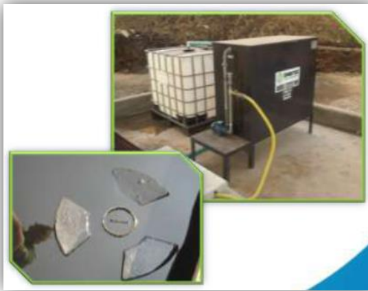
Figure 2-10 Photographs of an Oil/Water separator.
