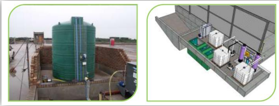
Figure 2-11 Photograph and illustration of a holding tank and closed circuit system.
