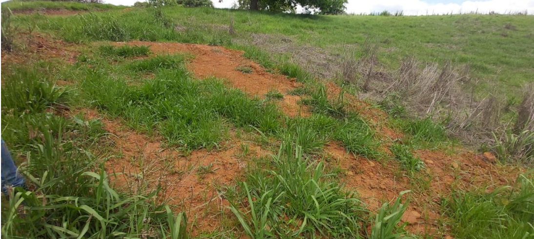
Figure 16: Plant kikuyu runners across the contours of the banks adjacent to the deck and stabilise with geojute and 'intengus' at 0.5 – 1m intervals
