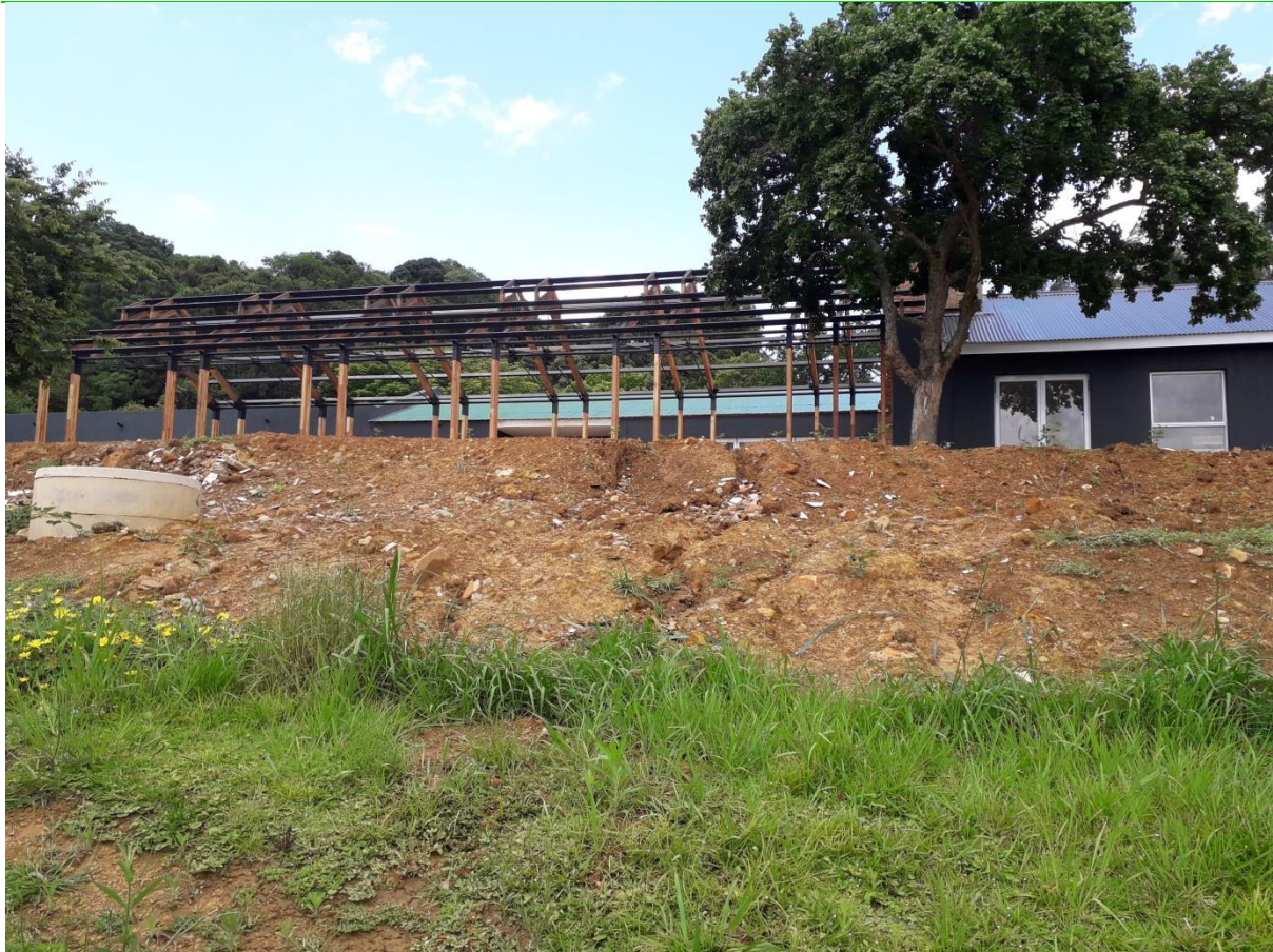
Figure 20: Clear rubble and use it to fill erosion channels. Smooth bank and plant with kikuyu runners across the contours of the banks at the main house and stabilise with geojute and 'intengus' at 0.5 – 1m intervals.
