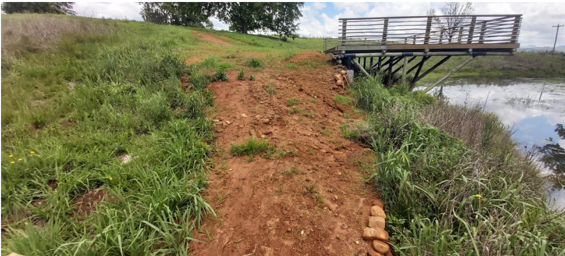
Figure 17: Terrace the pathway to a maximum width of 1.5m, using poles and surface with gravel. Plant kikuyu runners up to the pathways, across the contours and stabilise with geojute and 'intengus' at 0.5 – 1m intervals
