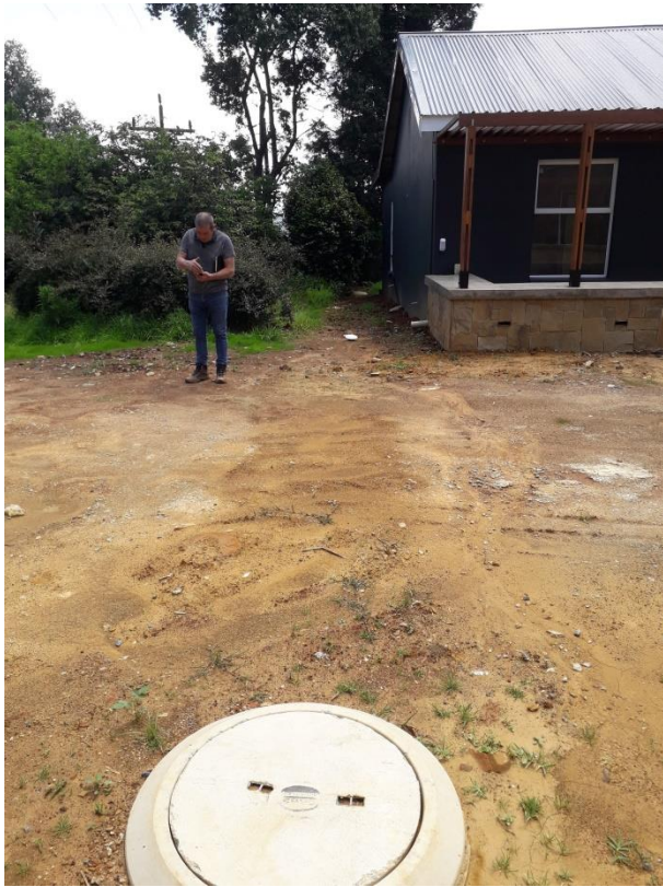
Figure 23: Seed the driveway areas with Cynodon dactylon and install waterbars/pole drains at an angle of about 10°, which will trap the silt, but turn and direct the water to the downhill side of the slope.
