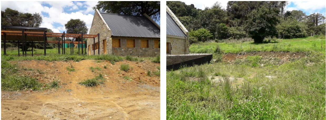
Figure 14: Plant kikuyu runners across the contours of the banks at the staff house/laundry and stabilise with geojute and 'intengus' at 0.5 – 1m intervals
