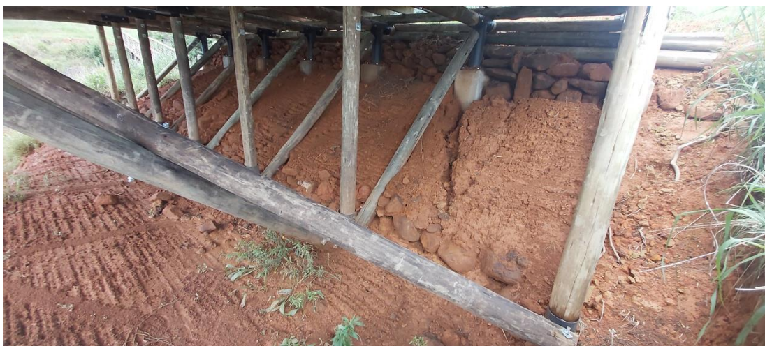
Figure 15: Install rock gabions in wire cages underneath the wooden deck
