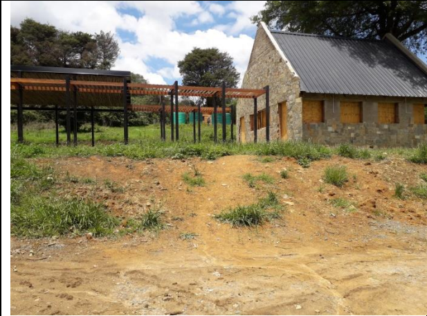
East towards laundry
