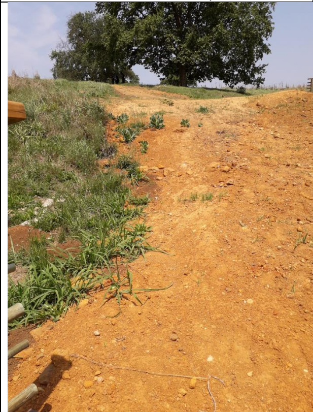
Walkway from bridge past wooden deck (south)
