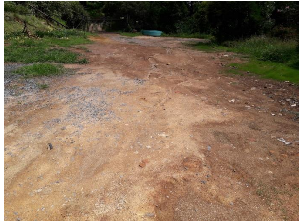
Figure 23: Seed the driveway areas with Cynodon dactylon and install waterbars/pole drains at an angle of about 10°, which will trap the silt, but turn and direct the water to the downhill side of the slope.
