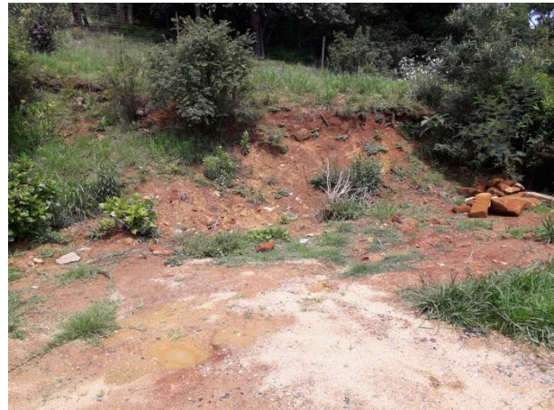
Figure 23: Seed the driveway areas with Cynodon dactylon and install waterbars/pole drains at an angle of about 10°, which will trap the silt, but turn and direct the water to the downhill side of the slope.
