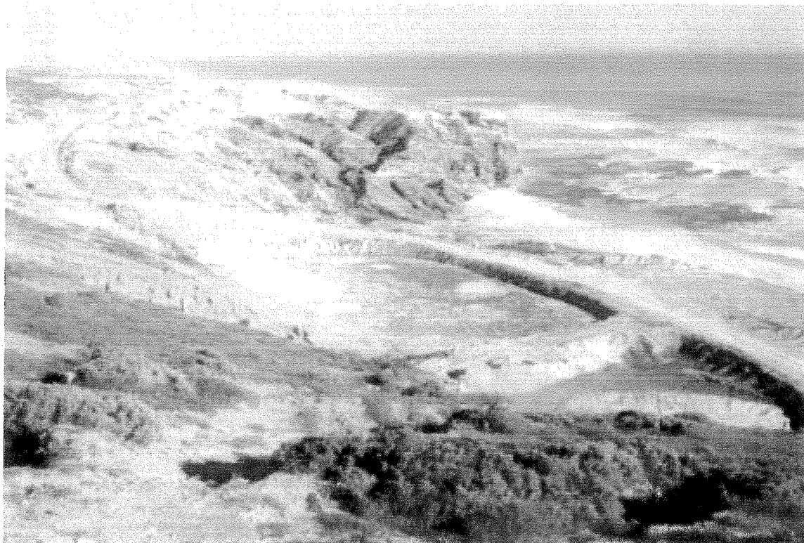
Plate 7: The slimes residue dams at the base of the cliff below the gravel processing plant. Fine materials from the diamond extraction process are pumped to this dam as a sediment slurry. The fines settle out and the clean seawater percolates back into the sea.
