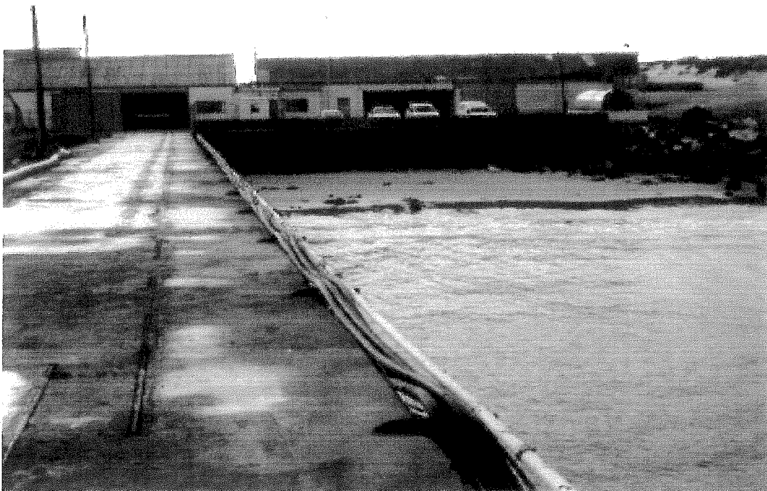
Plate 3: The Trans Hex gravel processing facility at . Workshops, offices and decompression facilities are located in the right-hand building and the processing plant in the left-hand building. Port Nolloth Security fence, fuel store and jetty approach are also shown.
