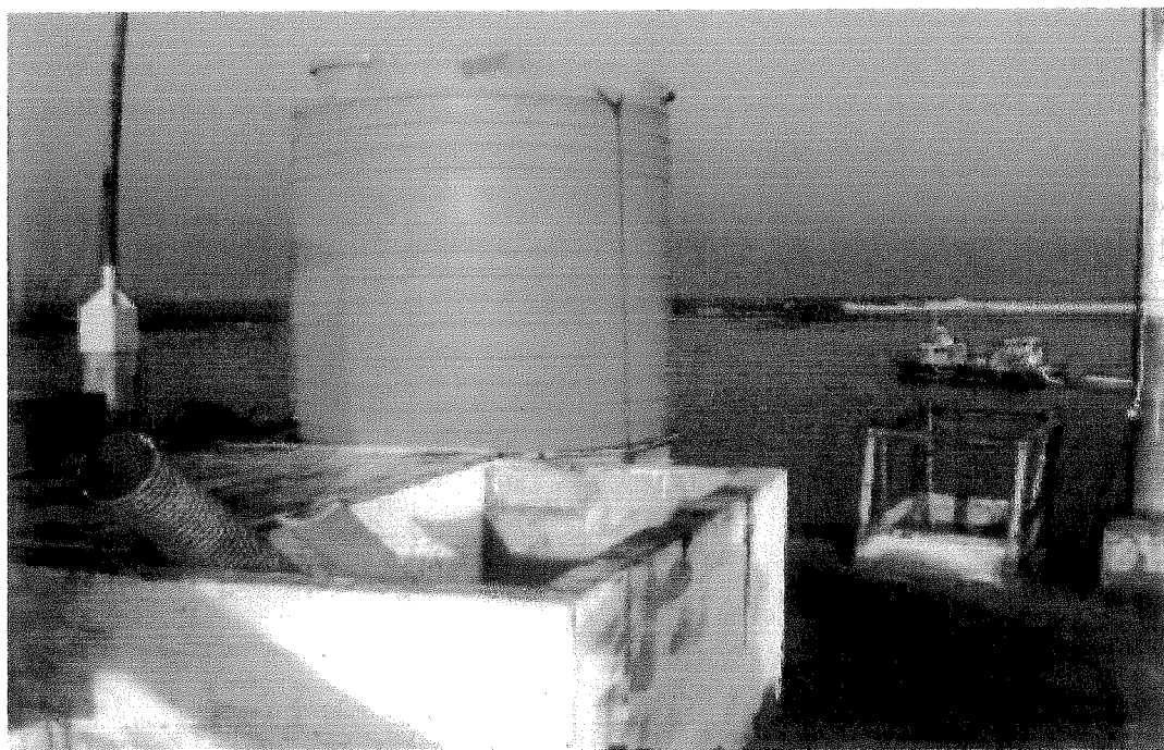
Plate 5. The water container and concrete skip on the Trans Hex jetty at Port Nolloth.
