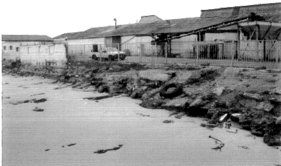
Plate 4: The Trans Hex gravel processing plant at Port Nolloth. The slimes dam is located behind the wall adjacent to the beach in the left of the photograph. Clean seawater from the dam percolates back onto the beach. Tailings are stored in the hoppers and frequently collected by building contractors.
