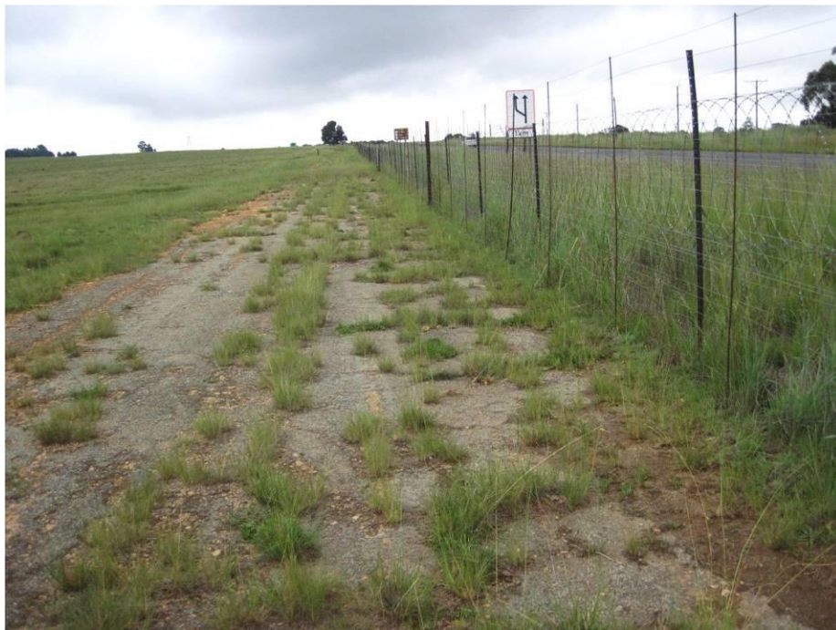
Figure 6: The security fence along the southern edge of the N4 motorway, with the remains of the erstwhile two-lane tar road to the Lowveld in the foreground.
