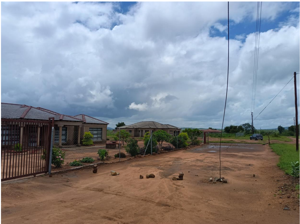
The existing powerlines and poles on site
