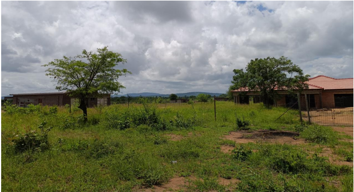
The other portion of houses with no electricity connection
