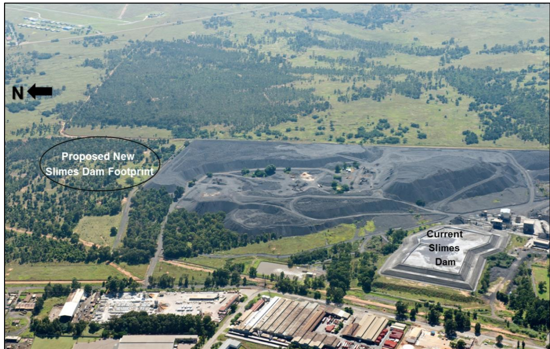
Figure 8.3.1(c): Best Alternative Footprint (new Slimes Dam) and Existing Slimes Dam Footprint
