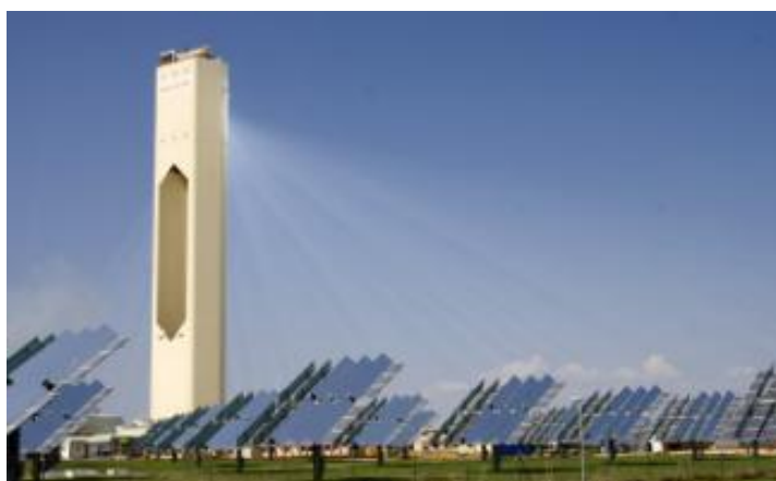
Figure 1-6: CSP in Seville, Andalusia, Spain
