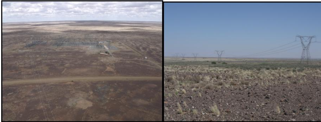
Figure 7-26: Bushmanland Basin Shrubland surrounding Aries substation
