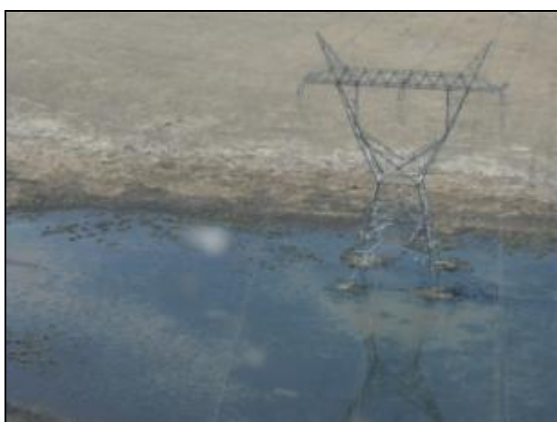
Figure 1-8: Example of a river crossing
