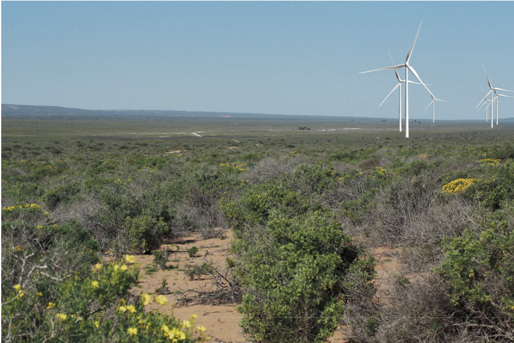
Figure 15: Photo simulation 3 (after construction). Distance to closest turbine = 6km.
