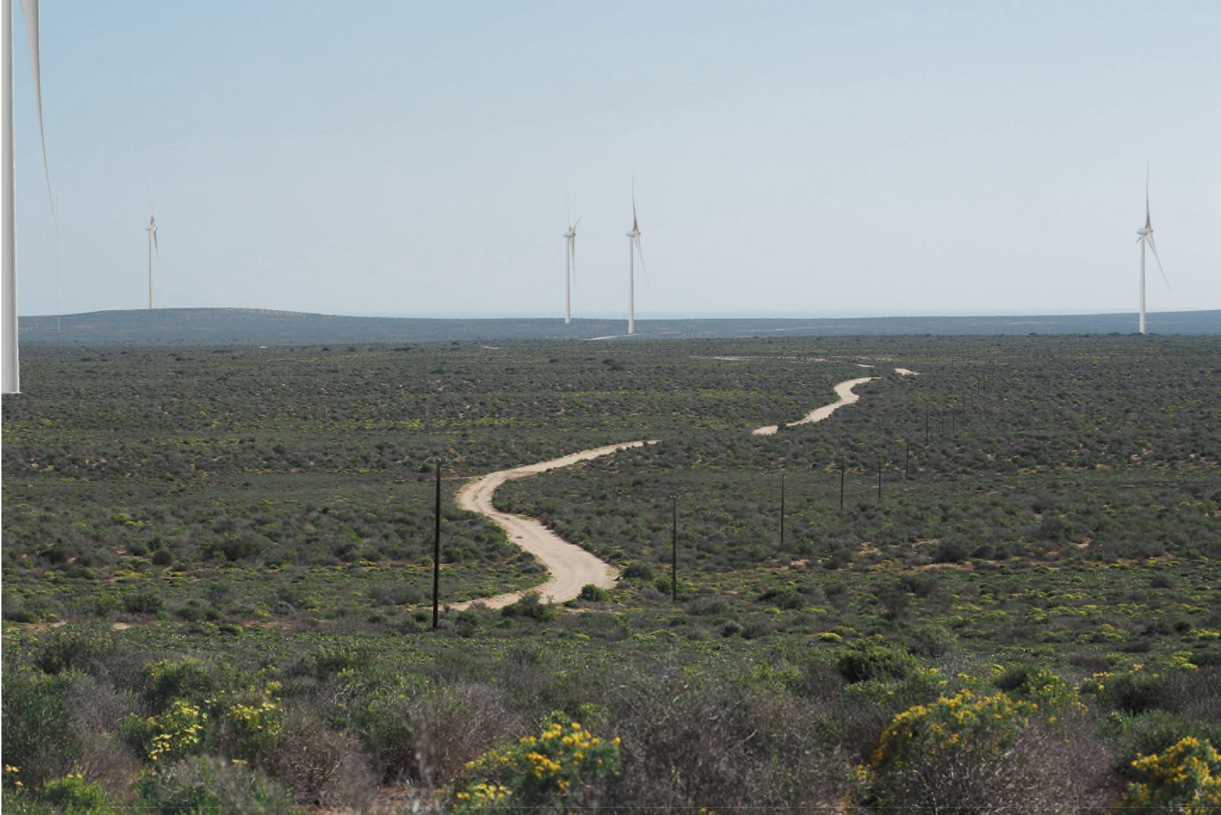
Figure 17: Photo simulation 4 (after construction). Distance to closest turbine = 3km.
