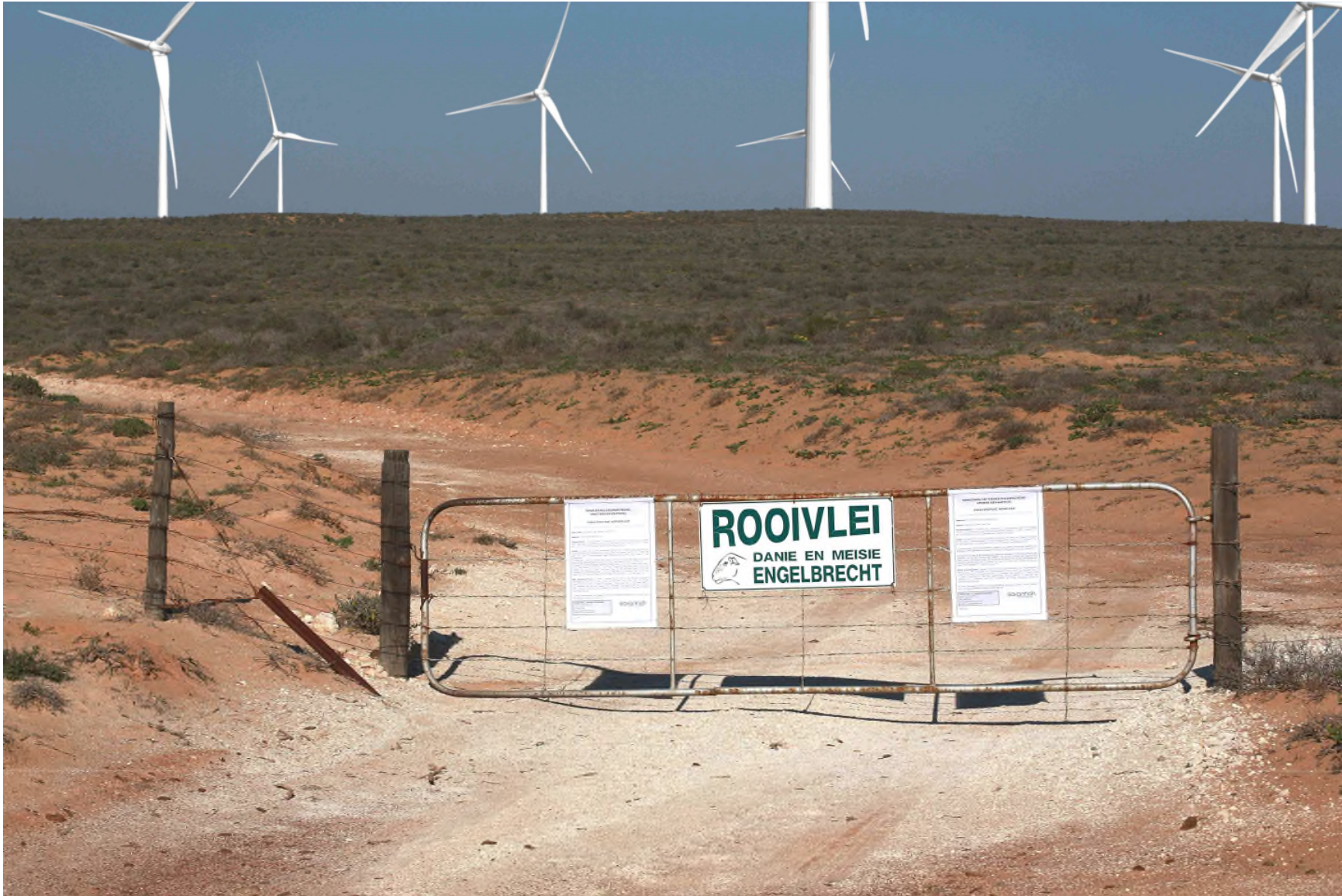
Figure 13: Photo simulation 2 (after construction). Distance to closest turbine = 1km.
