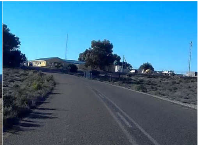
Photograph 2-12: MR751 Surfaced Section
