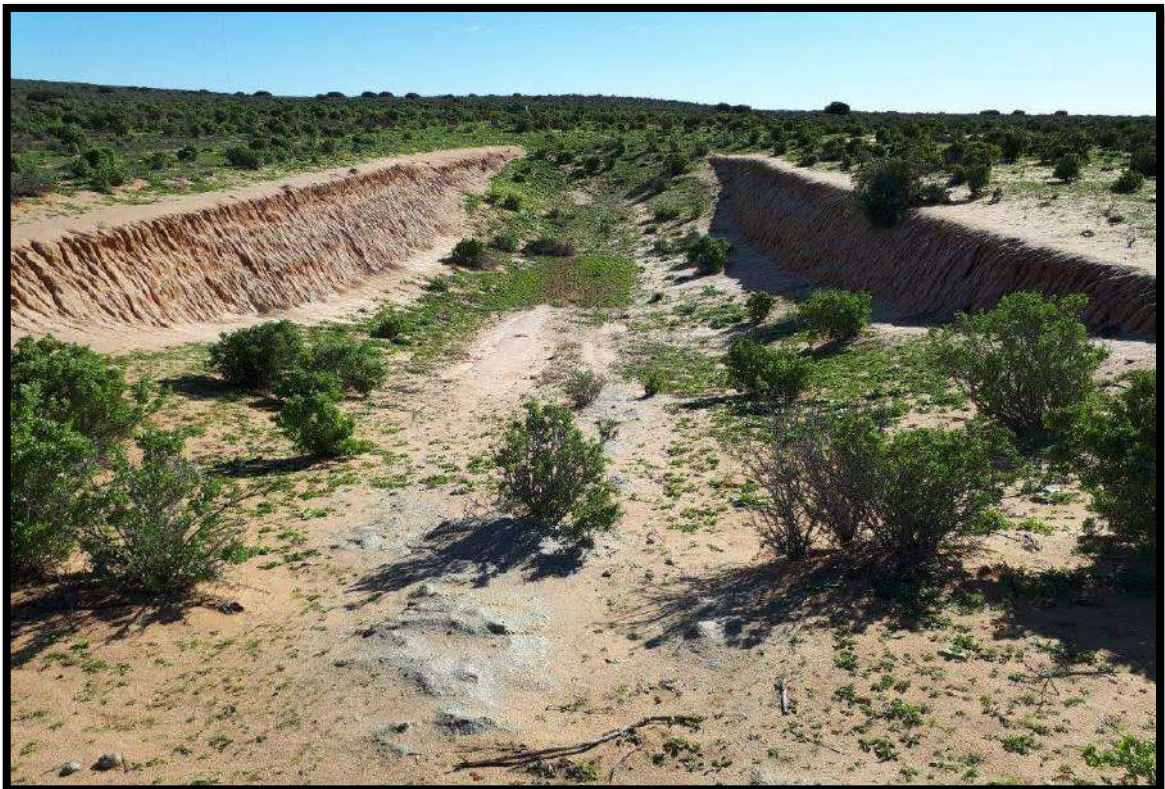
Figure 1-9 and Figure 1-10: Note the erosion damage at the man-made borrow pit areas. Note the reddish sand soils above and the whitish calcrete sand below. These depressions also serve as storm water detention ponds, to retain a storm water flood, in the event of abnormal high rainfall.
