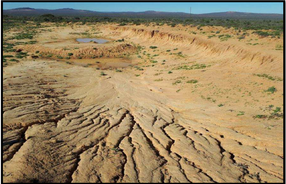
Figure 1-9 and Figure 1-10: Note the erosion damage at the man-made borrow pit areas. Note the reddish sand soils above and the whitish calcrete sand below. These depressions also serve as storm water detention ponds, to retain a storm water flood, in the event of abnormal high rainfall.
