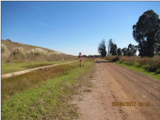
Figure 8: View of road and ditch in servitude of Ash Dam
