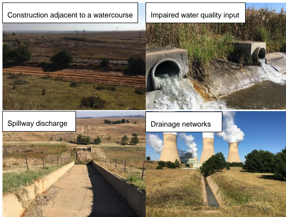
Figure 7: Photographic evidence of current general impacts observed on site
