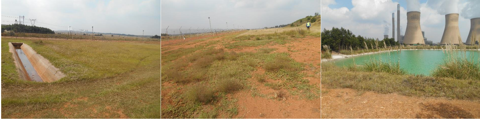
Figure 5: Photos of the High Level Dam Servitude
