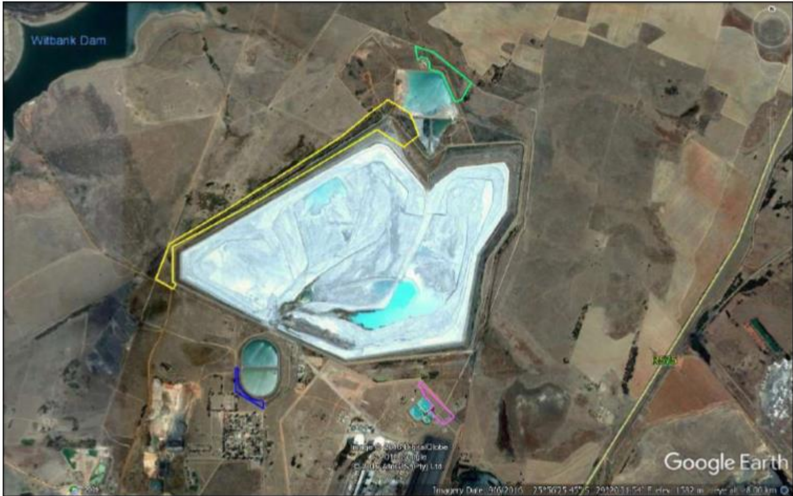
Figure 2: Google Earth image indicating the proposed servitude footprint areas for the seepage interception drains (blue, green, pink and yellow polygons) (Map provided by Nemai Consulting).
