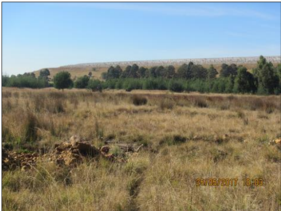
Figure 6: View of Ash Dam from outside the servitude north-western boundary
