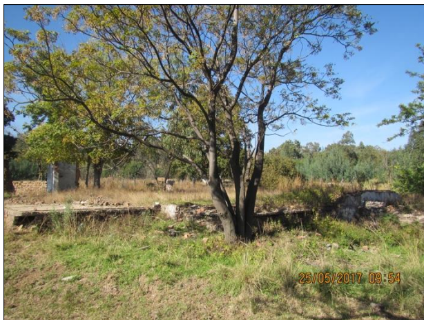
Figure 22: View of DUV001, showing the foundation of one of the buildings
