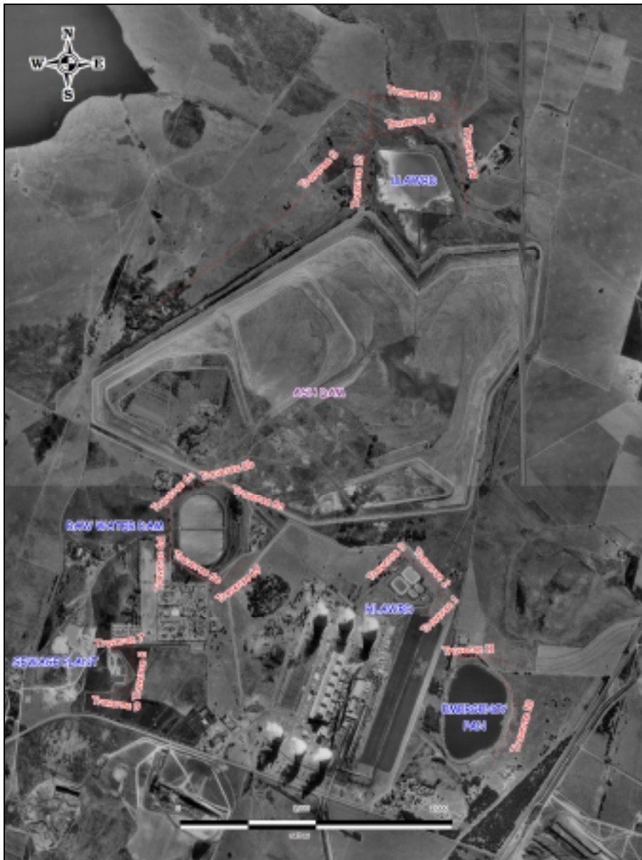
Figure 8. Positions and orientations of the magnetic traverses in relation to the dam systems at Duvha Power Station.
