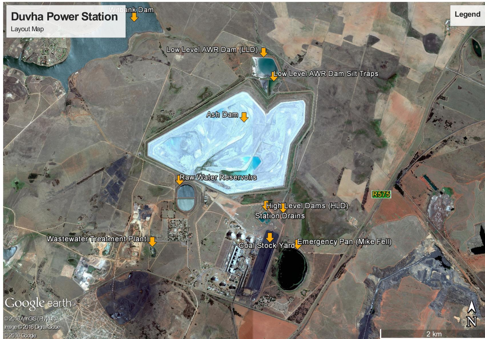
Figure 2: Layout of Duvha Power Station
