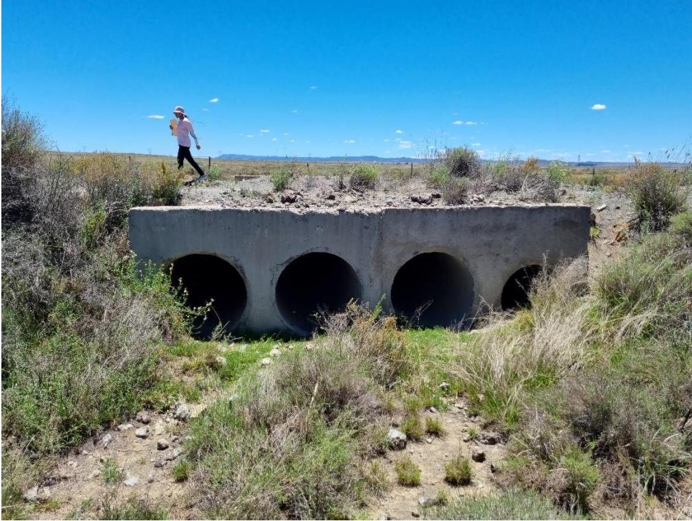
Photo 5: Existing pipe culvert on the public district road section (facing Northwest).
