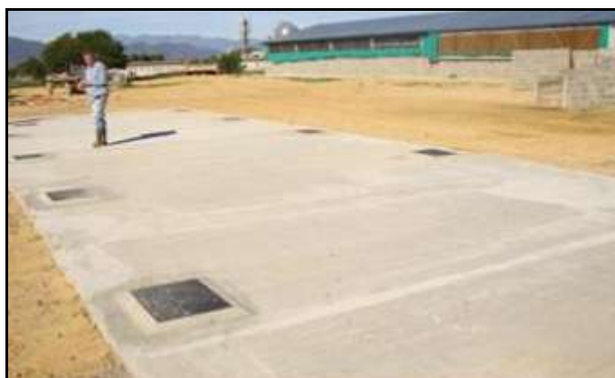
Photo 7.8: An example of a concrete sump with lid (provided by Big Dutchman, 2017)
