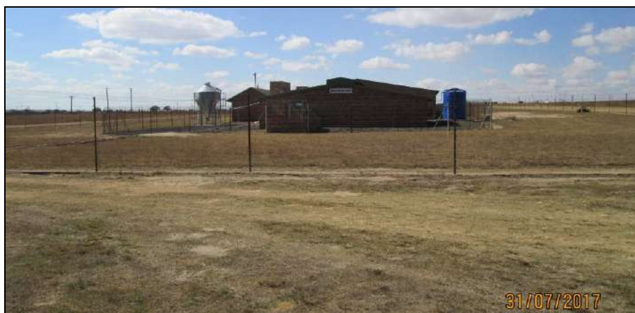
Photo 3.1: A view of the existing GTC facility located on the farm Rockdale.
