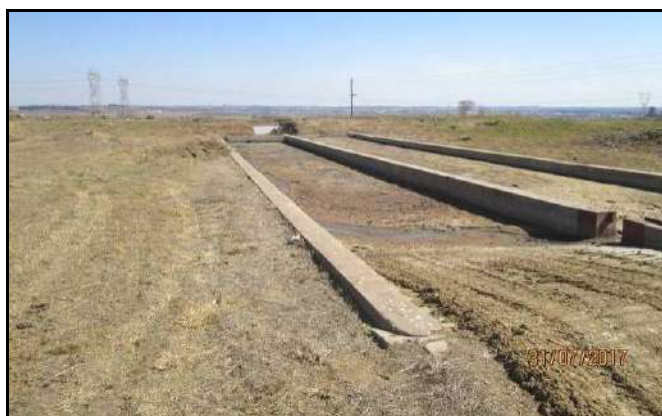
Photo 7.3: A view of the two evaporation manure pits at the existing GTC facility.
