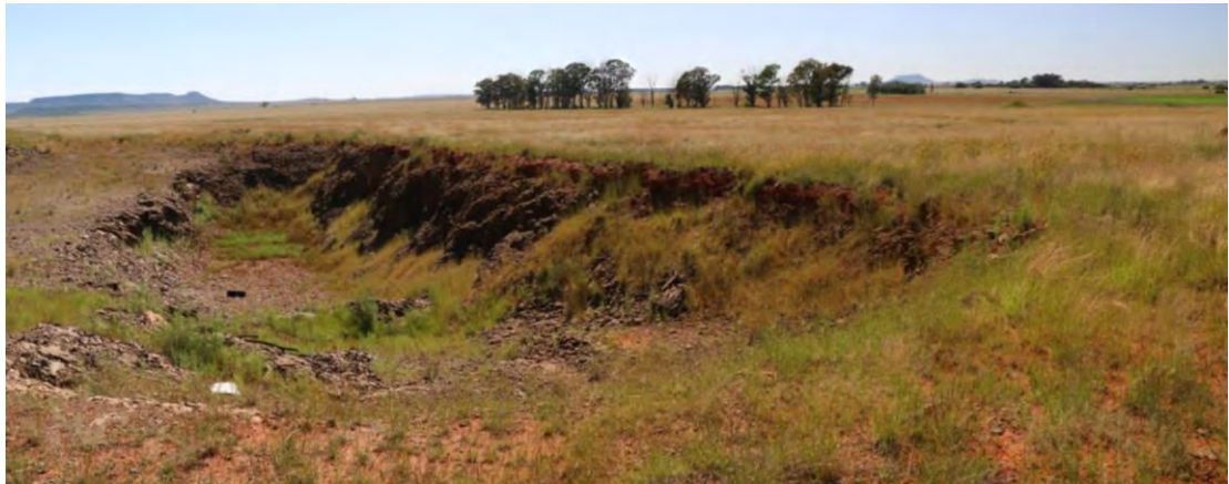
Figure 2: Panorama of the site showing the existing borrow pit excavation. Note that it remains free draining.
