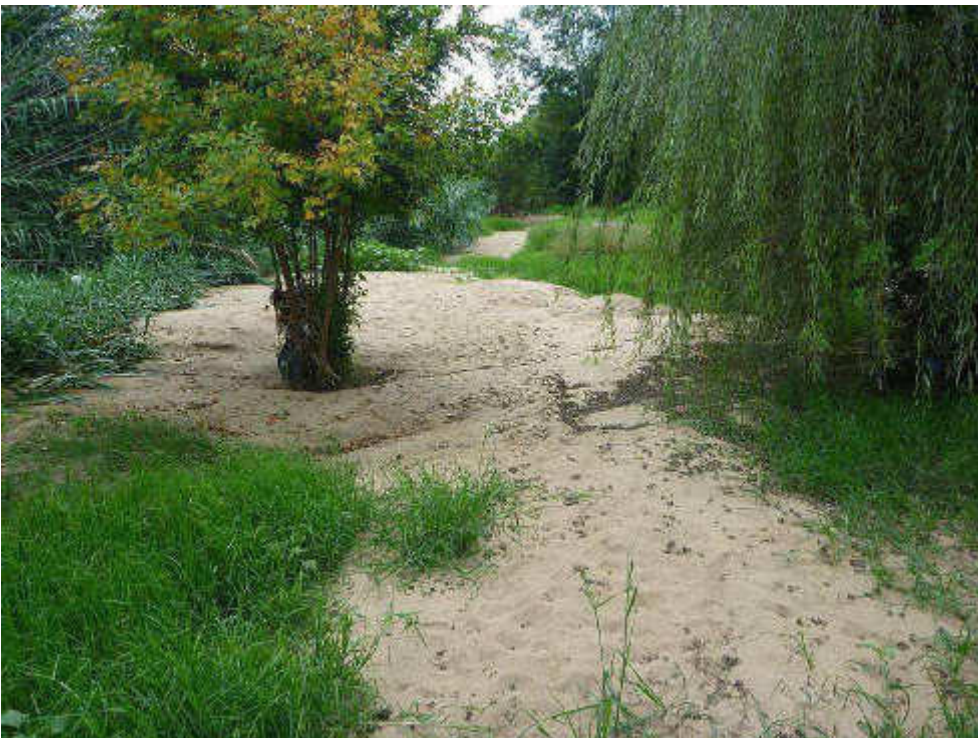
Figure 18 Significant sedimentation (of granitic origin from upstream of the survey site) within the drainage channel the Rietspruit near the end of Poole Avenue
