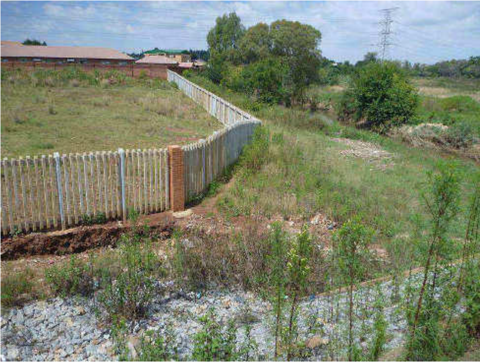
Figure 13 Fence and gabion structures on the banks of the Rietspruit at the R55 river crossing (eastern side)
