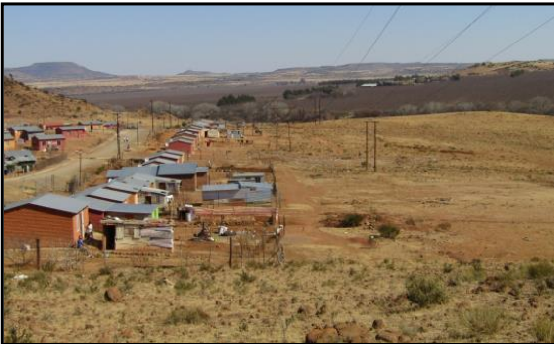
Photo 11: Location of Existing 66kV and 22kV in relation to Area 13, Dukathole
