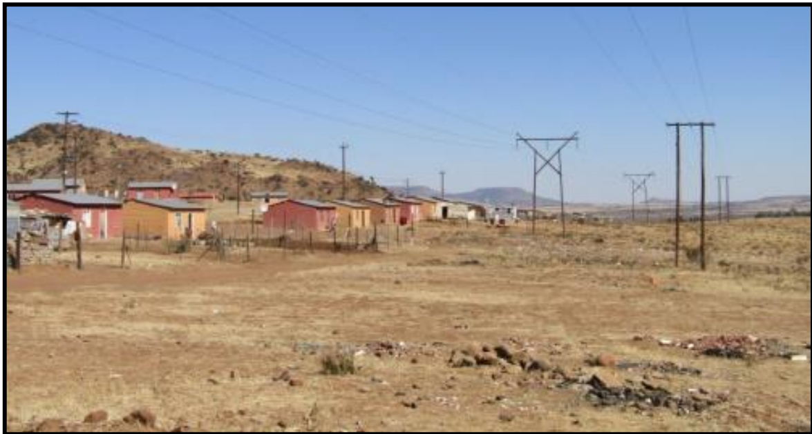
Photo 3: View of the existing power-lines near Area 13, Dukathole
