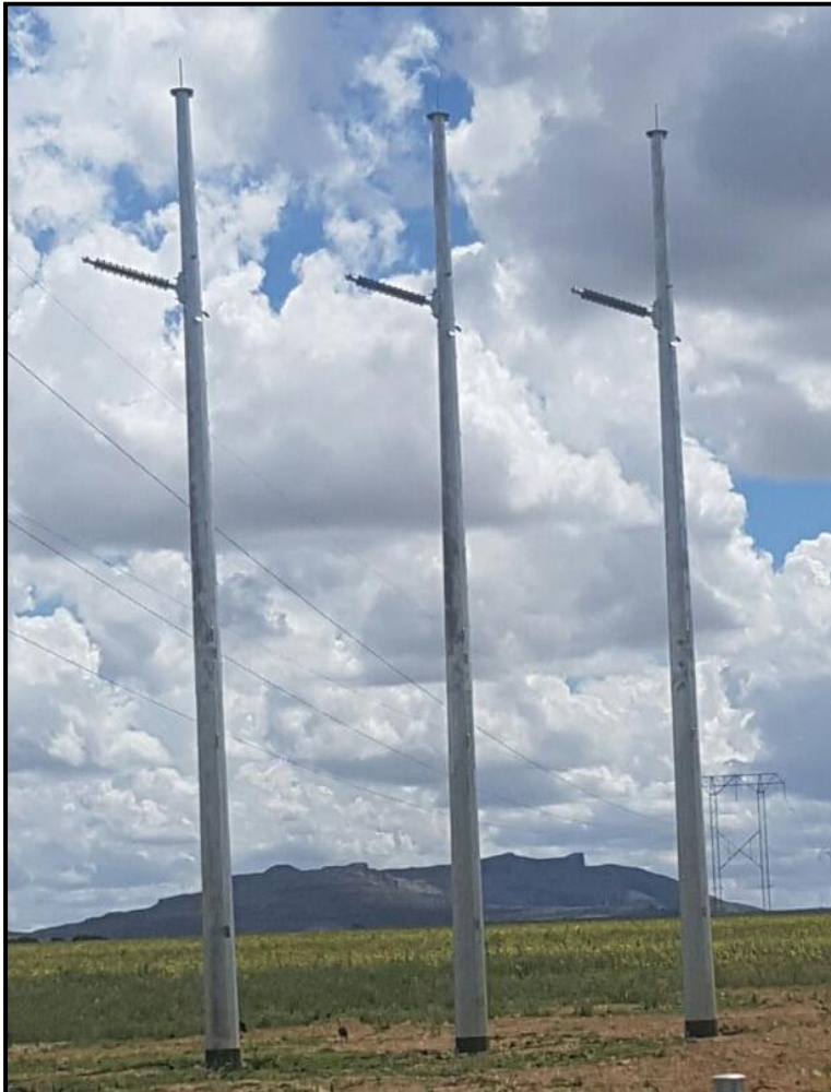
Figure 1: Picture of a Monopole Tower
