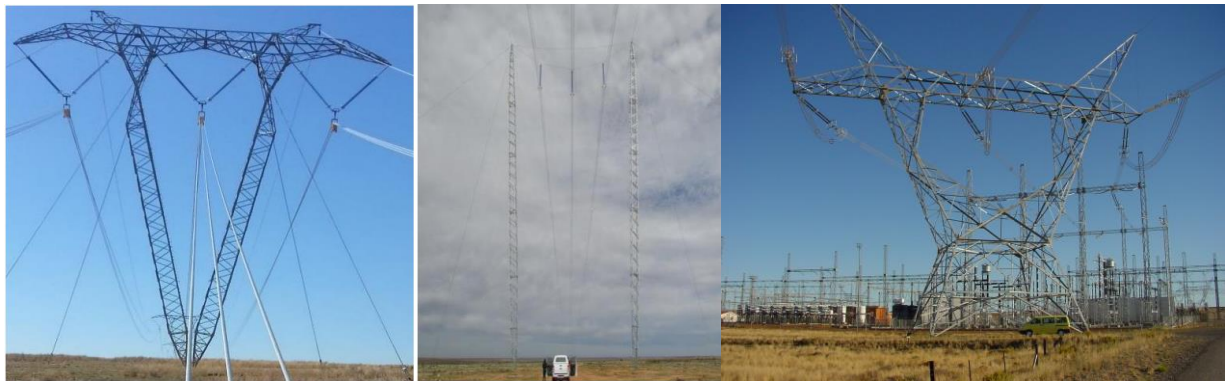
Figure 4-3: Typical 400kV Guyed V type (left) and Cross-Rope suspension (middle) and self-supporting (right) design
