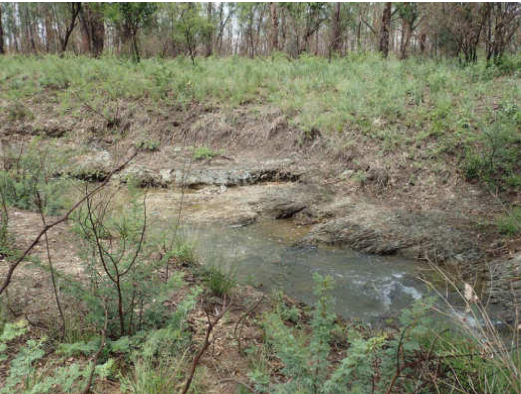
Figure 29 Eroded channel along the watercourse
