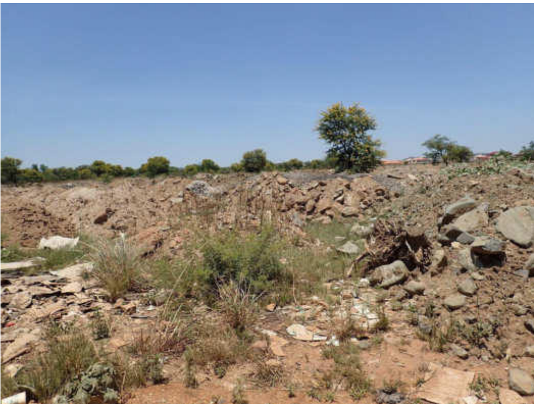
Figure 17 Dumping of rubble on the site
