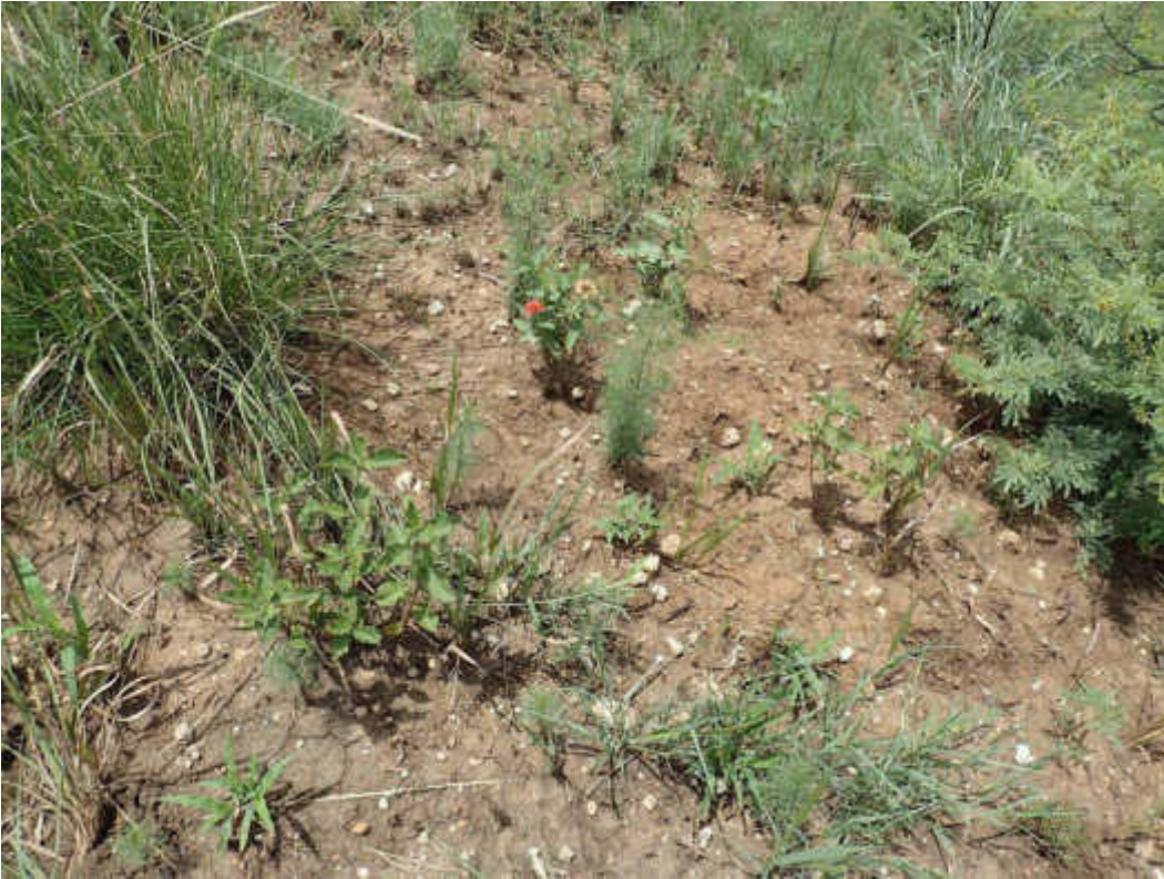
Figure 30 Exposed lime nodules in a subsoil horizon with surface horizons removed through erosion along the watercourse
