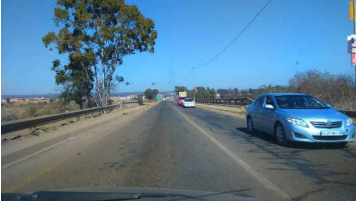
e) Bridge crossing looking south on the M10
