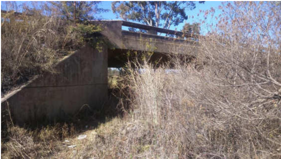
f) Bridge crossing
