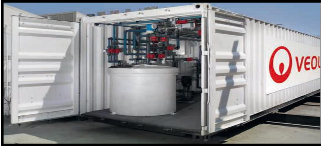
Fig6: Proposed Containerised Sewer Treatment Plant
