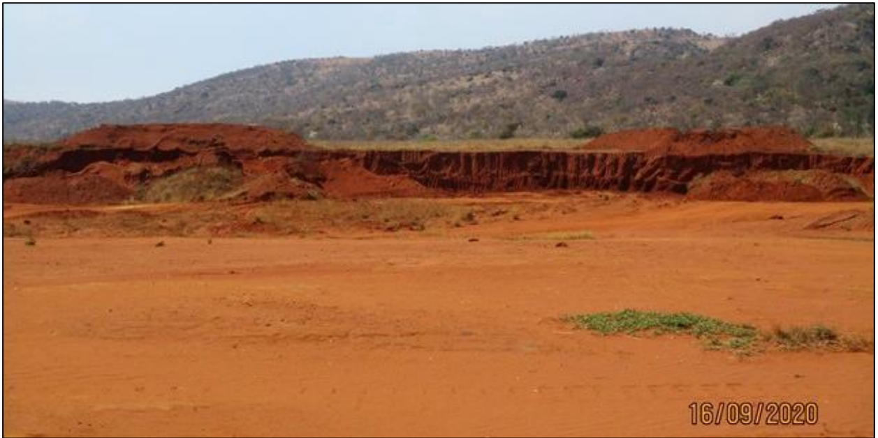
Photo 2: Example of excavations.
