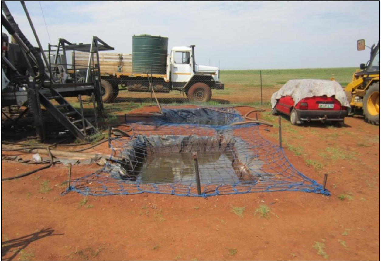
Photograph 2: Indication of the sumps required for a typical drilling operation.
