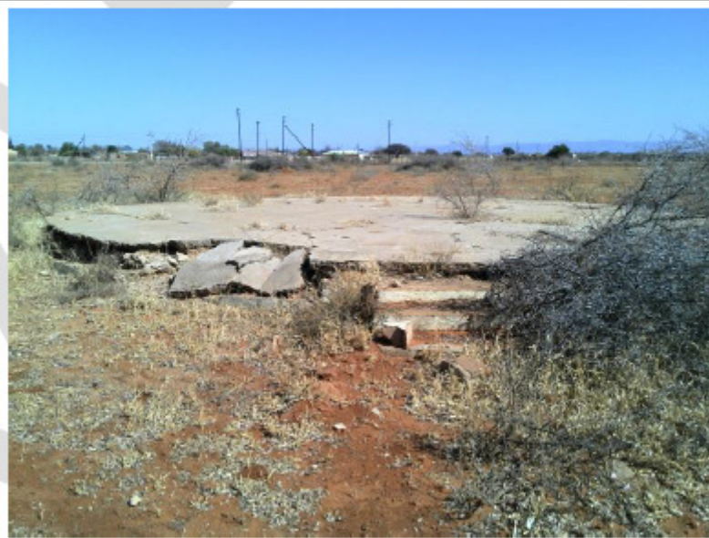
Figure 18: Cement foundation in the study area
