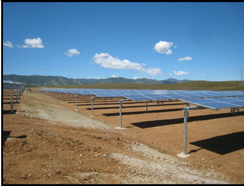
Figure 2-4: Example of a single axis tracking system with PV arrays arranged in parallel (courtesy: Mulilo)
