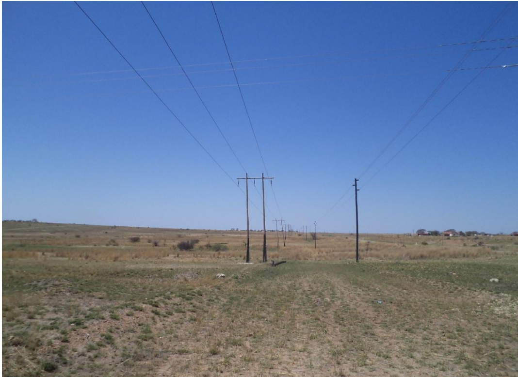
Fig. 8: shows the current wooden poles used for the proposed powerline
