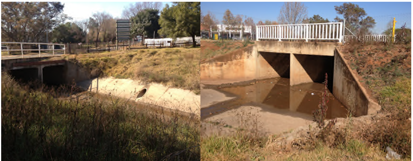
Culverts and Bridges on Sonja Street and Jasper Avenue Respectively
