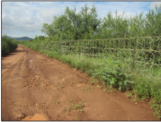
Plate 1 :Gravel access road and razor-wire boundary fence
