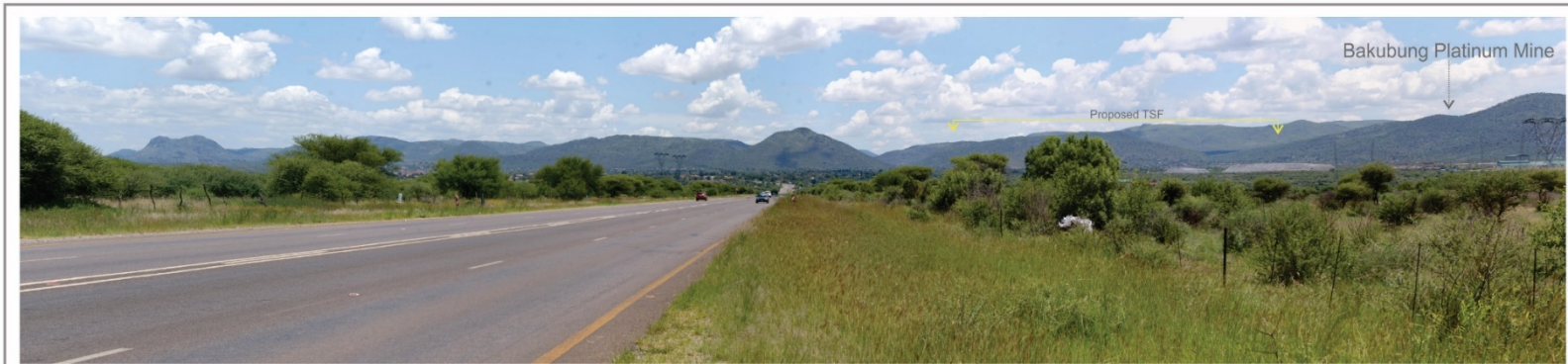
View 4: From a local road (R565), approximately 2.5km south of the proposed TSF site.
