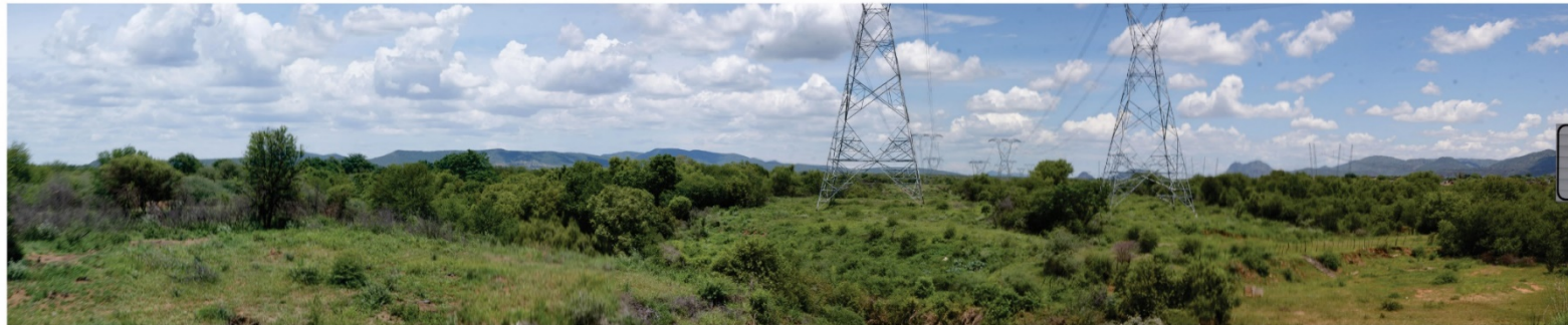
View of the Authorised TFS site, photo taken from the Elandriver Bridge (R565).
