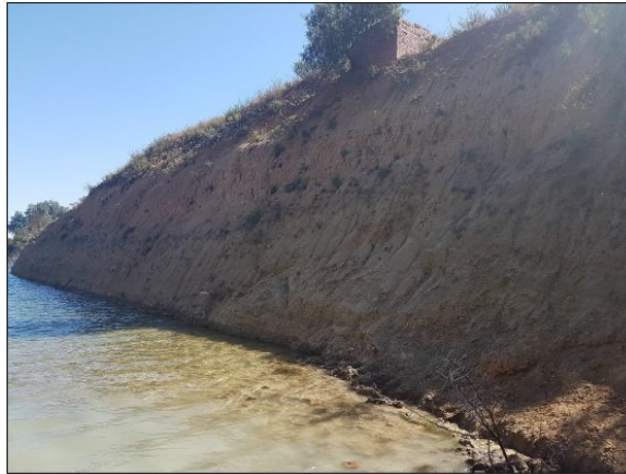
FIGURE 24: PHOTOGRAPHS SHOWING THE SOIL PROFILE OF THE QUARRY DAM WALL SOUTH OF THE PROPOSED SITE.
