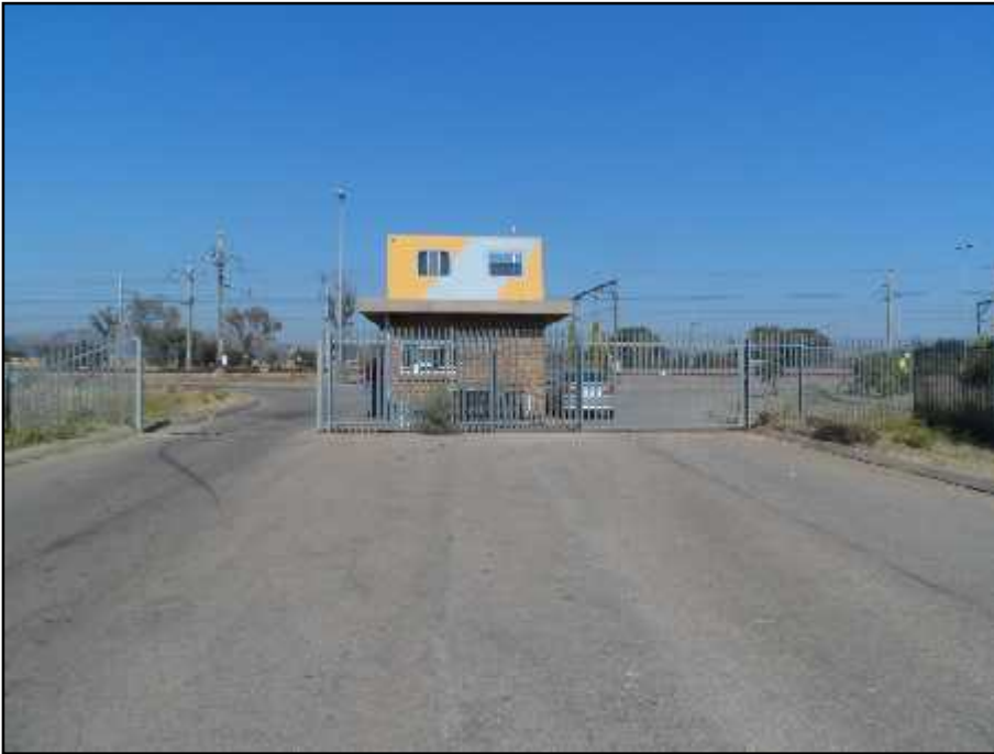
Figure 16-Existing Wolmerton guard house/security check point
