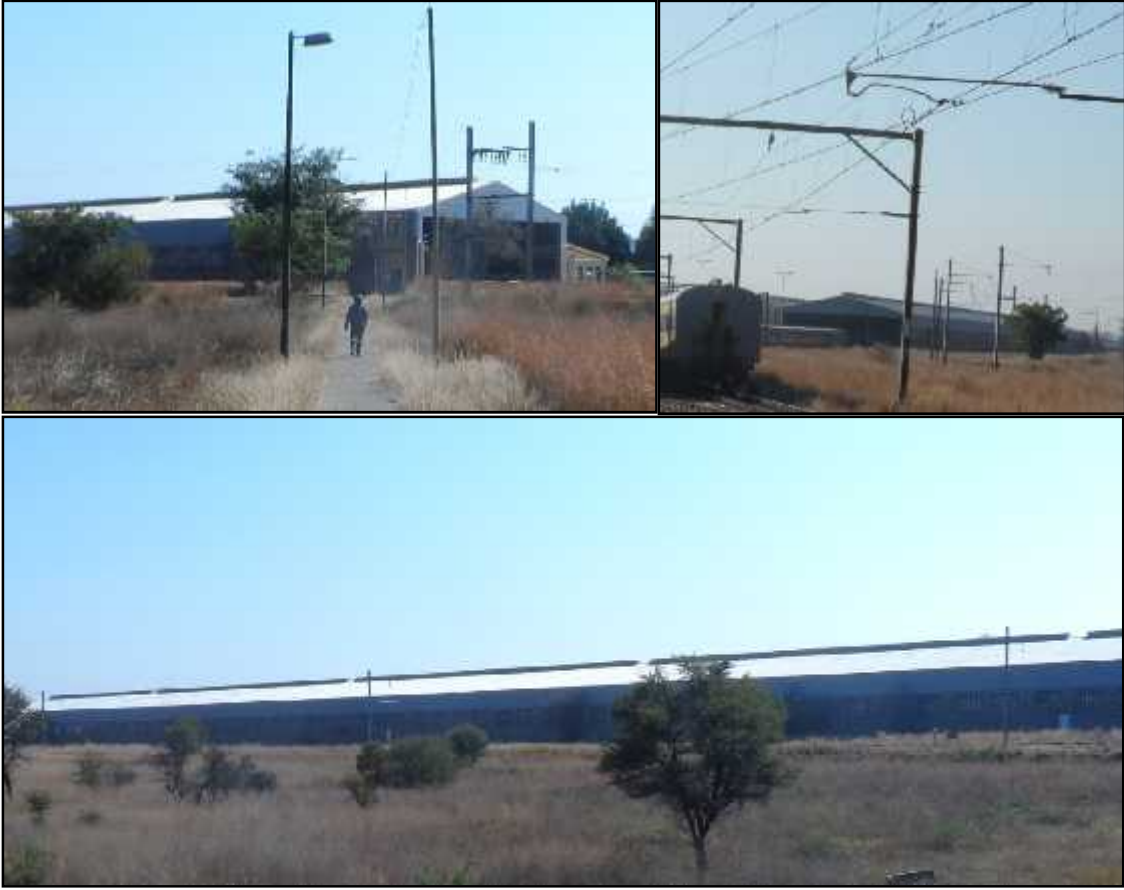
Figure 14- Existing Wolmerton running shed
