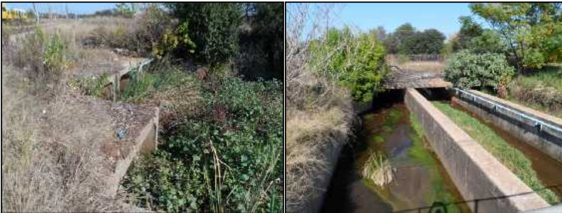
Figure 6 - Storm water infrastructure
