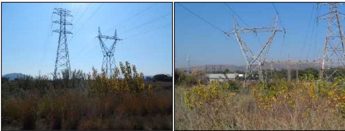
Figure 4- Eskom Transmission Lines (cross the site) and a Substation on the south-eastern tip of the site
