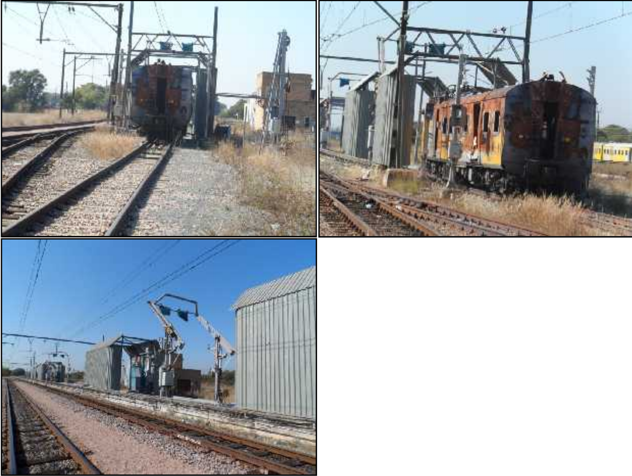
Figure 15- Existing Wolmerton external automated washer
