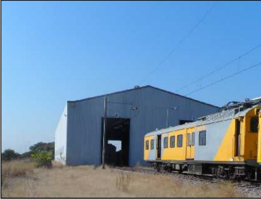
Figure 13- Existing Wolmerton lifting shop
