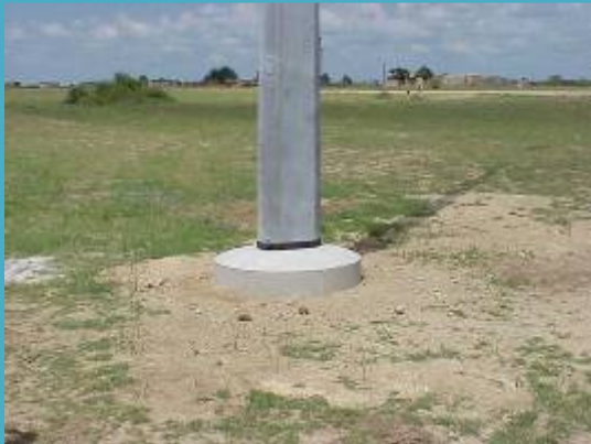
Figure 5. Foundation excavation (source: Eskom)
