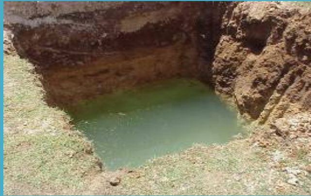
Figure 4. Foundation excavation (source: Eskom)
