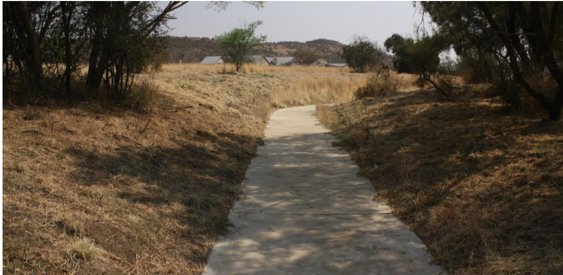
Figure 9: View of the drainage line downstream of the site where it has been canalised. It is recommended that the proposed development incorporate it in much the same manner.
