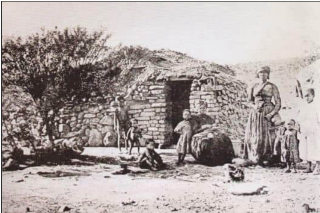
Figure 7-83: A shepherd's hut photographed near Beaufort West in the early 20th century. Note the low, narrow doorway and informal roof structure. Source: Schoeman (2013:48)
