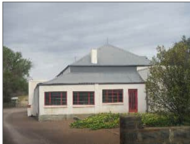
Figure 7-101: Historical structure at Slangfontein (waypoint 1747 in HL01)
