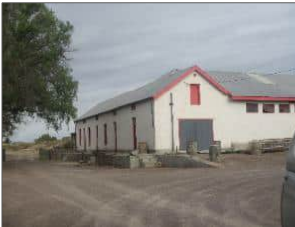
Figure 7-100: Historical structure at Slangfontein (waypoint 1747 in HL01)
