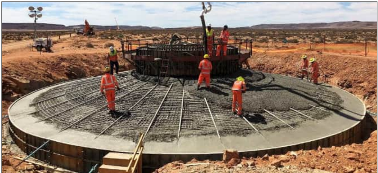
Figure 2-9: Example of a typical turbine foundation under construction
