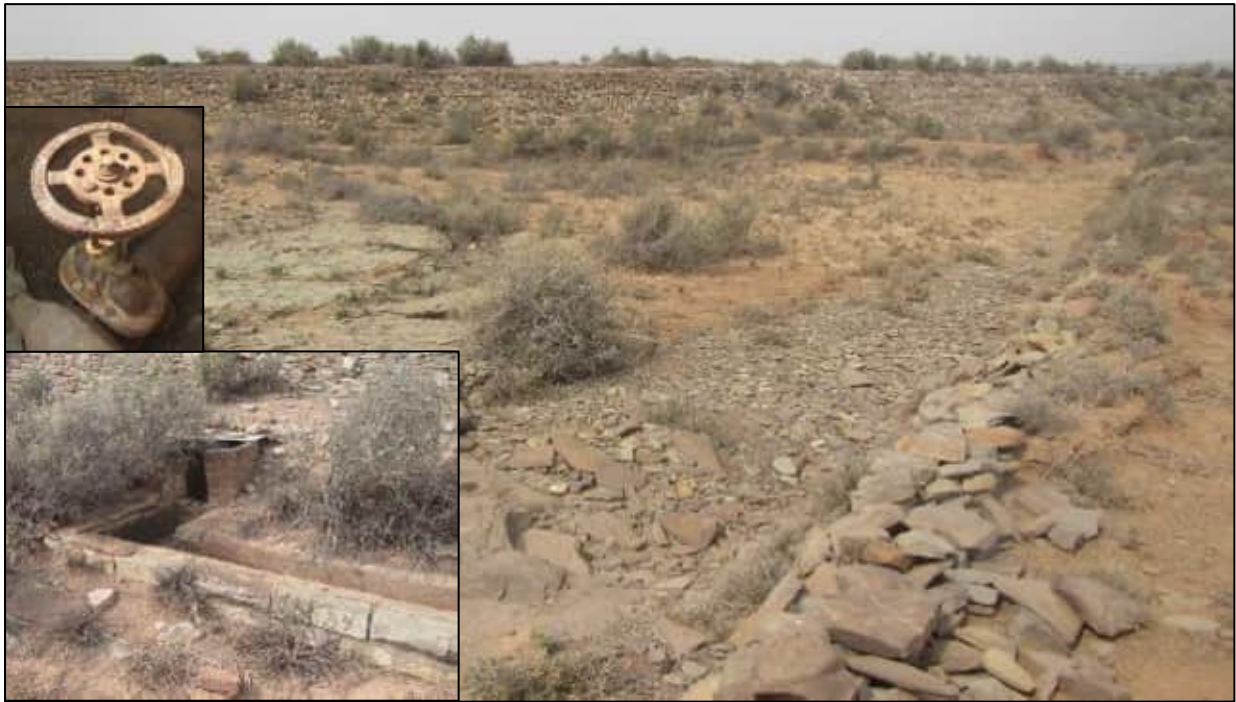
Figure 7-88: View of the large dam at waypoint 100 in HL02 with the insets showing the outlet valve and associated leivater
