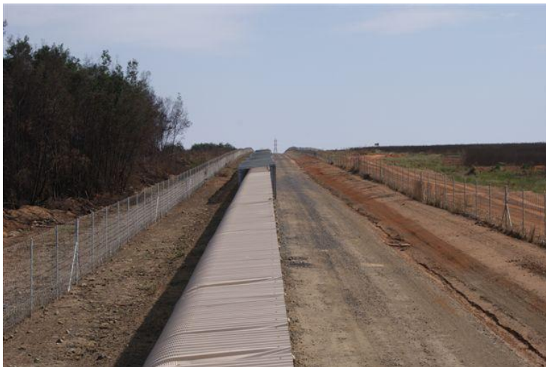
Plate 3-6: Typical example of a fenced servitude with conveyor belt and service road
