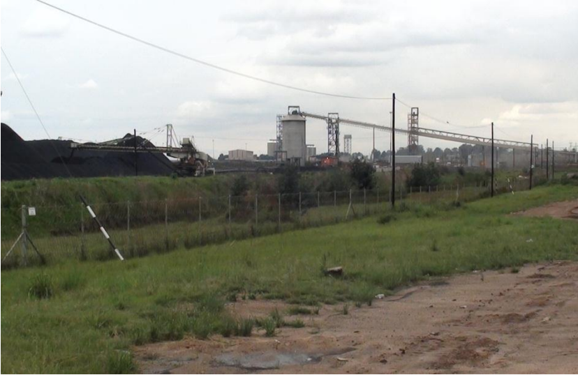
Plate 1-2: Phola Coal Processing Plant (CONVEYOR START POINT)
