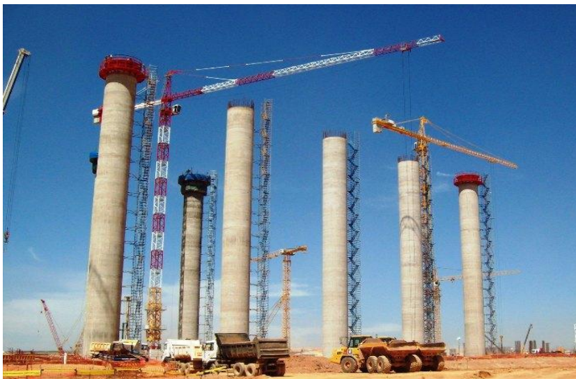
Plate 1-1: Kusile Power Station under construction (January 2010) (CONVEYOR DESTINATION)
