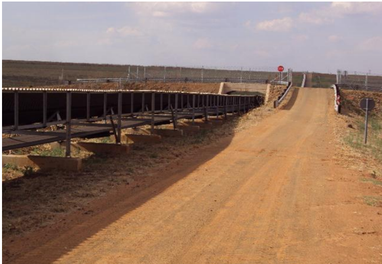
Plate 3-5: Example of a typical farm road crossing over conveyor
