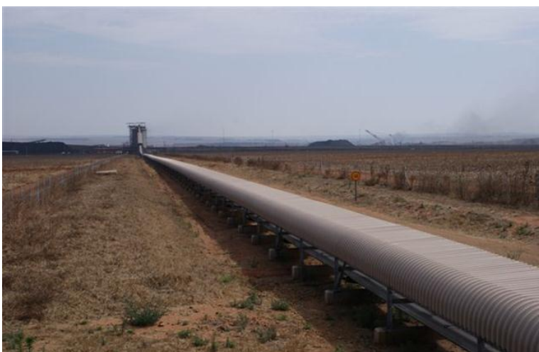
Plate 3-4: Example of a typical metal cover for conveyor belt
