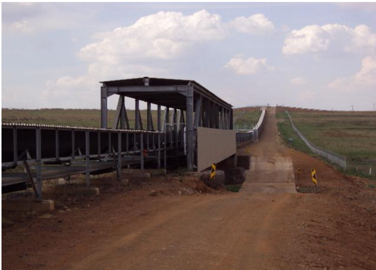
Plate 3-3: Example of a typical stream crossing with impermeable floor
