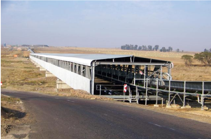
Plate 3-2: Example of typical wetland crossing (conveyor suspended on pillars, covered and with solid floor for collection of coal spills)
