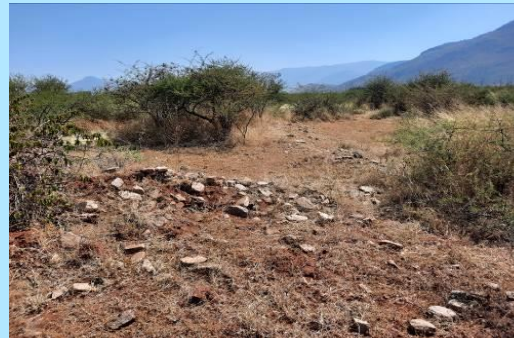
Figure 8-31: A series of broken-down structures and foundations
