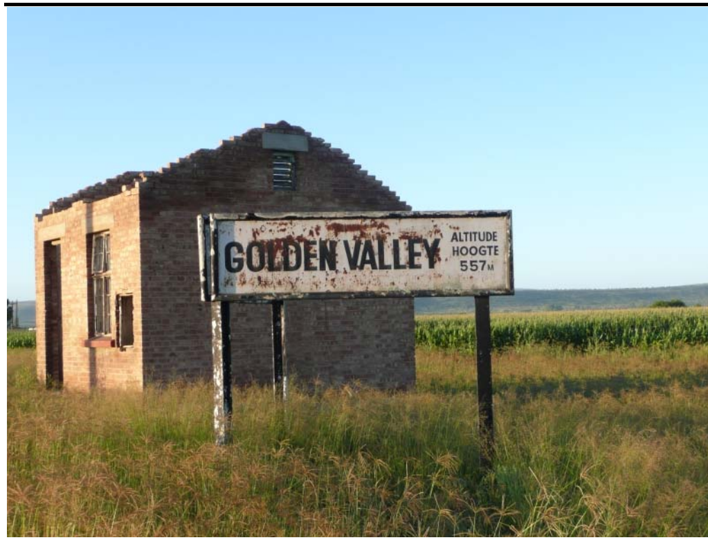
Figure 5.10 Abandoned station building at Golden Valley, Eastern Cape
