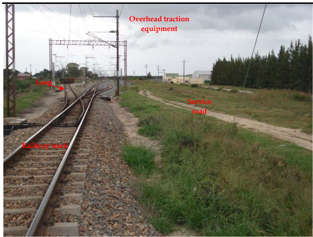
Figure 4.1 Existing loop to be extended at Barkly Bridge, Eastern Cape
