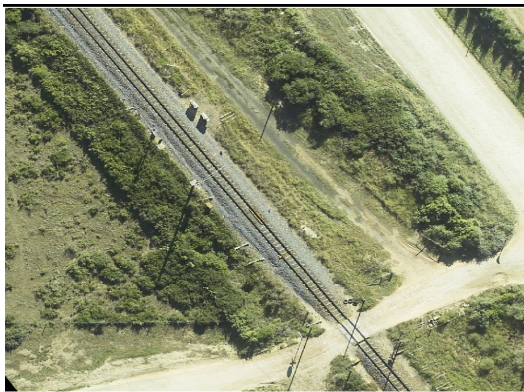
Figure 4.2 Aerial photograph of level crossing to be moved at Barkly Bridge
