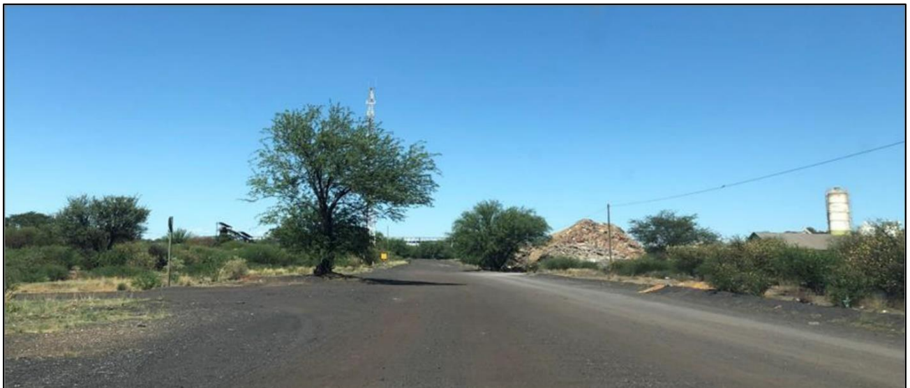
Figure 35: Proposed main entrance access road to the west of the mine
