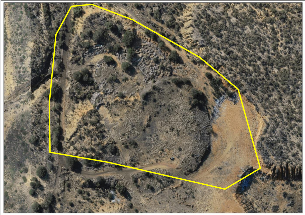
Figure 38: Google Earth Imagery of the Hotazel waste site located within the proposed THM
