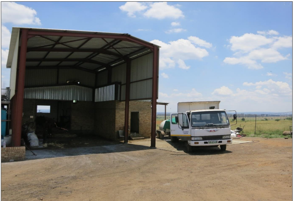
Figure 10: The waste intake area
