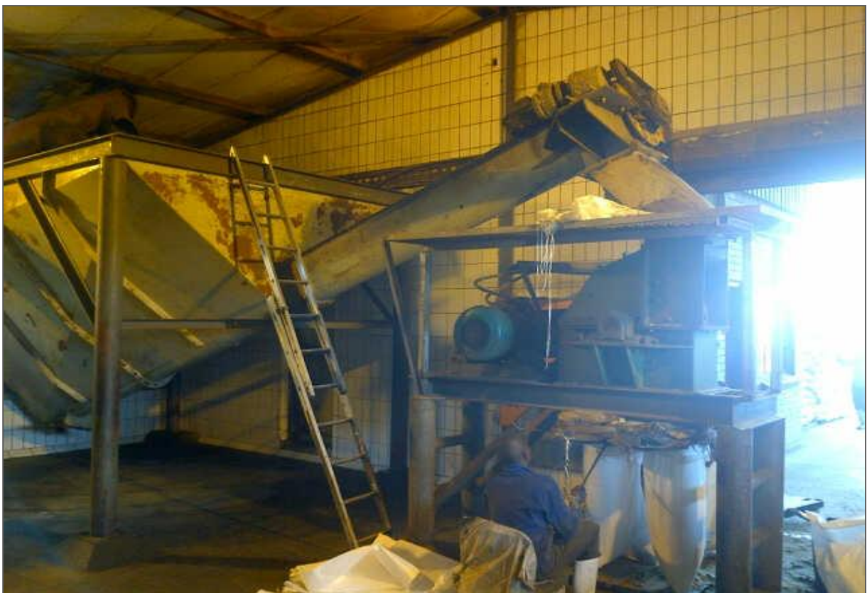
Figure 14: The bagging area
