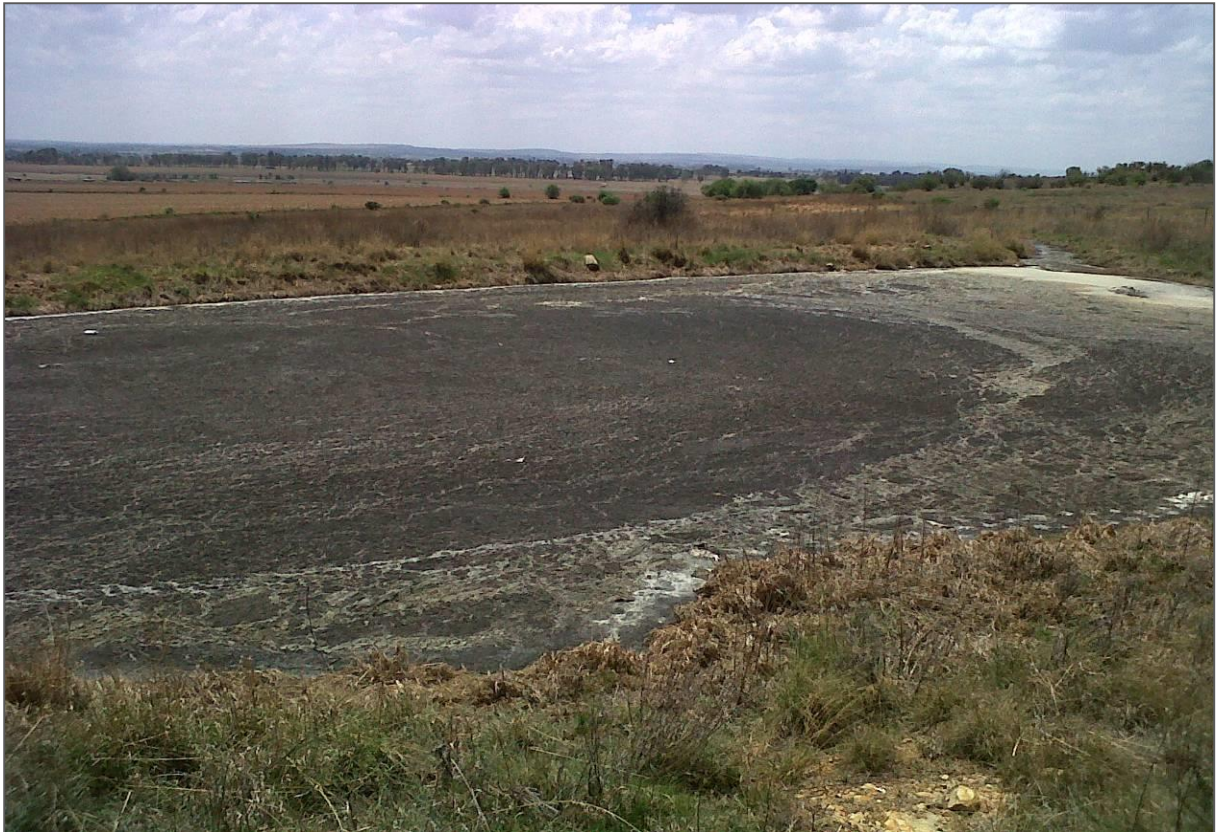
Figure 17: The existing wastewater evaporation pond
