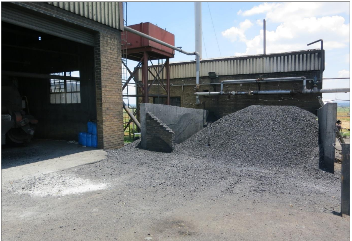
Figure 6: The coal storage bunker
