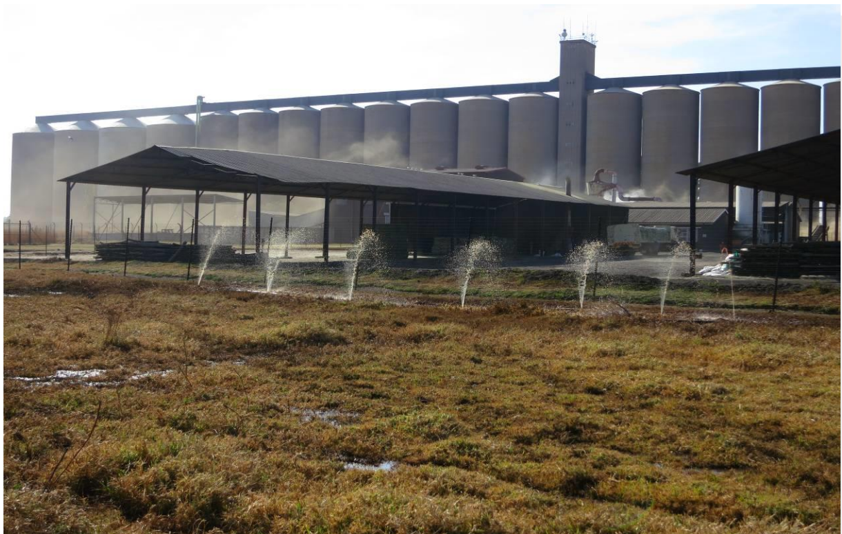
Figure 29: Wastewater from the settling pond is currently released into the environment (through irrigation) to the west of the rendering facility
