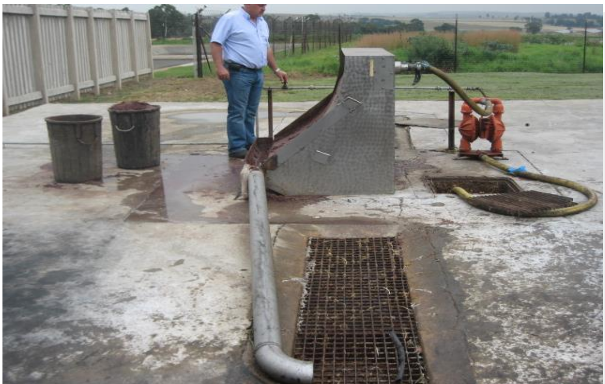
Figure 17: The wastewater collection sump and press (pre-filtration). Solids from the press are taken back to the storage bunker
