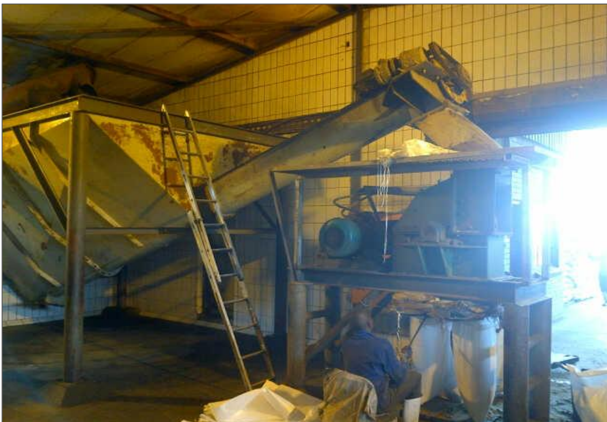
Figure 14: The bagging area
