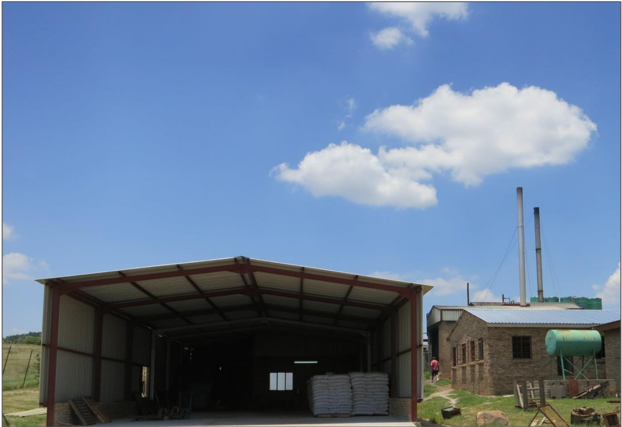
Figure 3: View of the rendering facility from the North-west
