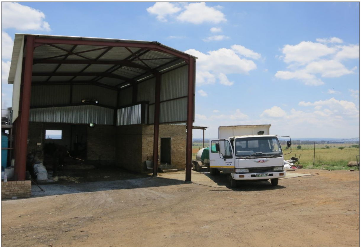
Figure 10: The waste intake area
