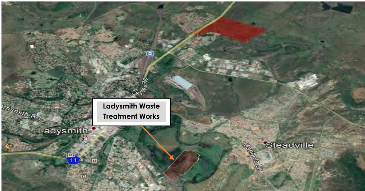
Figure 14 – Existing Waste Treatment Plant on site
