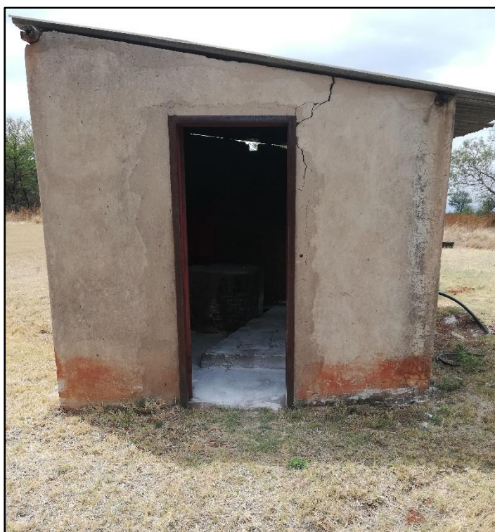
Figure 16. BULBH3 located within the pumping house.
