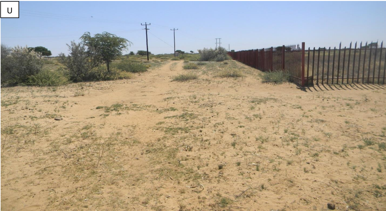
Plate 21 U: View of the 4 th T-off point for the proposed MV line.
