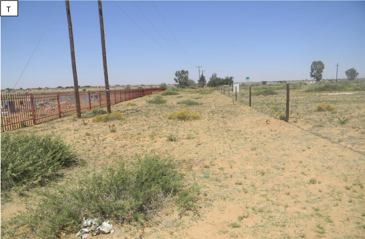
Plate 20 T: View of the 4 th T-off point for the proposed MV line.
