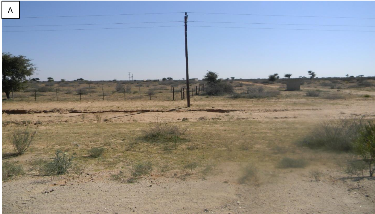
Plate 1A: View of T-off position for the MV line.
