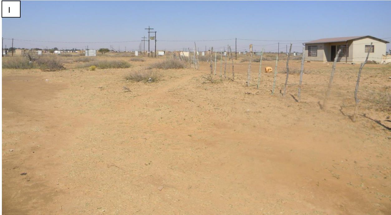
Plate 9 I: View of the T-off point for the proposed MV line from an existing transformer.
