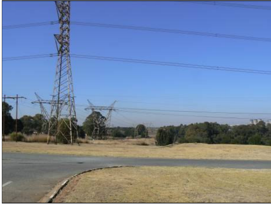
FIGURE 8: Existing power lines (route 3) between North Rand substation and Esther Park
