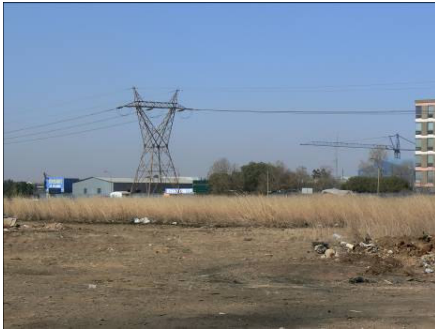
FIGURE 10: Existing power lines south of Edleen (route 3)
