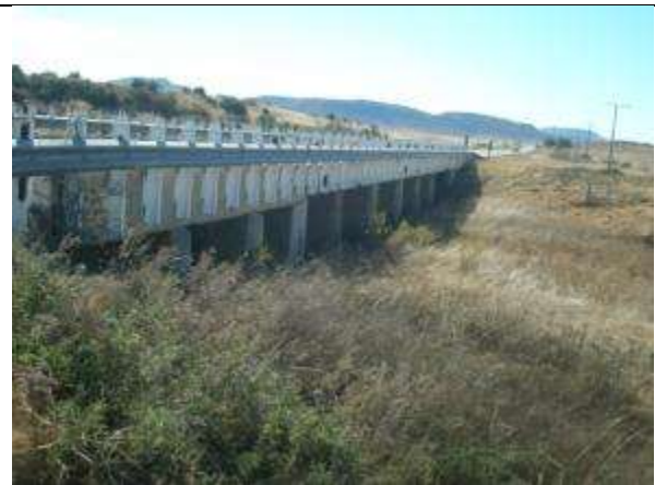
Elandskloof Spruit bridge: Widen/replace the existing bridge to suit new road alignment and cross section.
