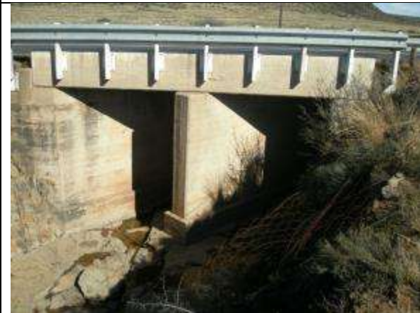
Wolwekop Stream bridge: Widen/replace the existing bridge to suit new road alignment and cross section. Capacity improvements.
