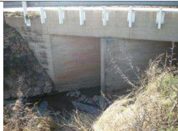
Wolwekop Stream bridge: Widen/replace the existing bridge to suit new road alignment and cross section. Capacity improvements.
