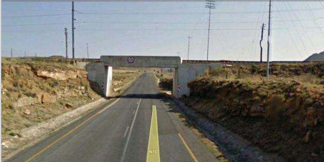
Photo of the Flonkers rail over road bridge that will be upgraded.
