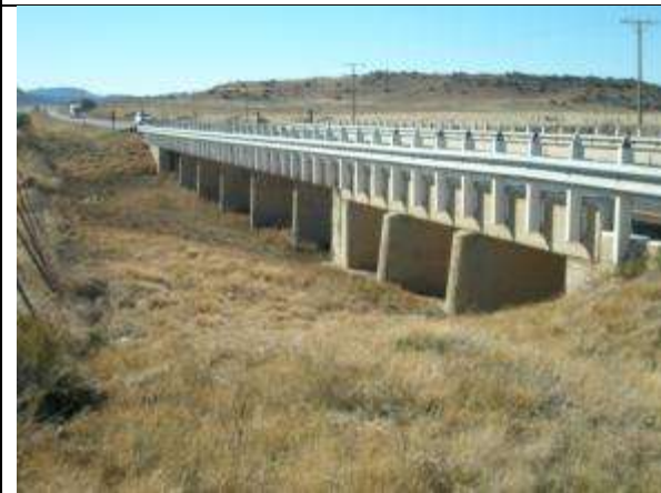
Elandskloof Spruit bridge: Widen/replace the existing bridge to suit new road alignment and cross section.
