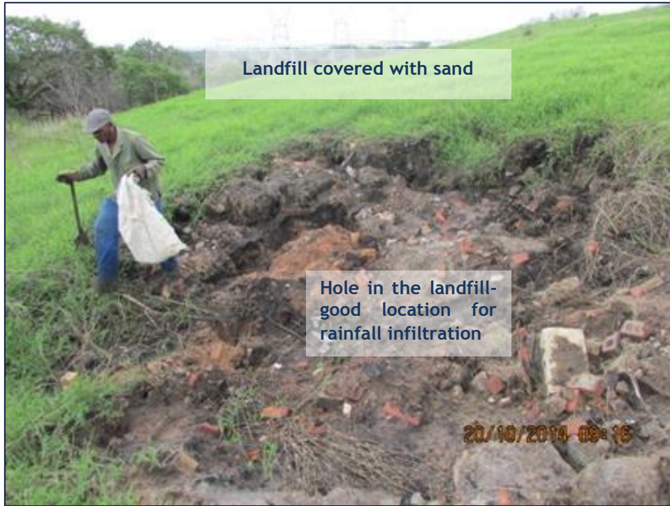
Figure 8-3: Photo showing a hole in the landfill and a man searching for steel
