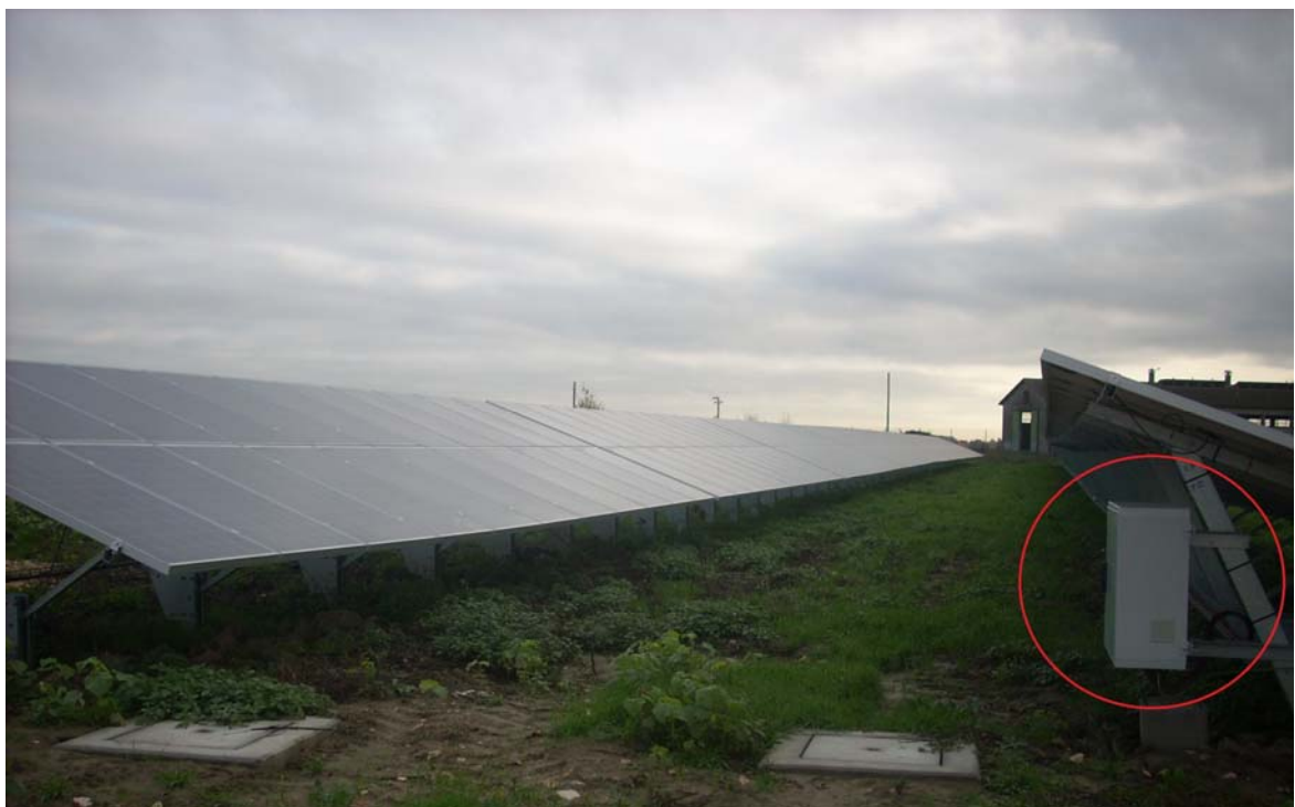
➤ Figure 10: A photo of a string box (red circle).
