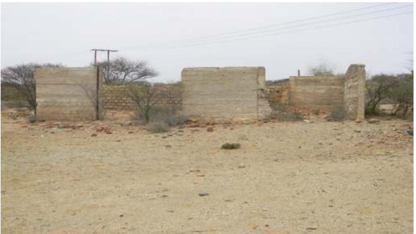
Figure 23: View of abandoned farm house within the proposed prospecting site
