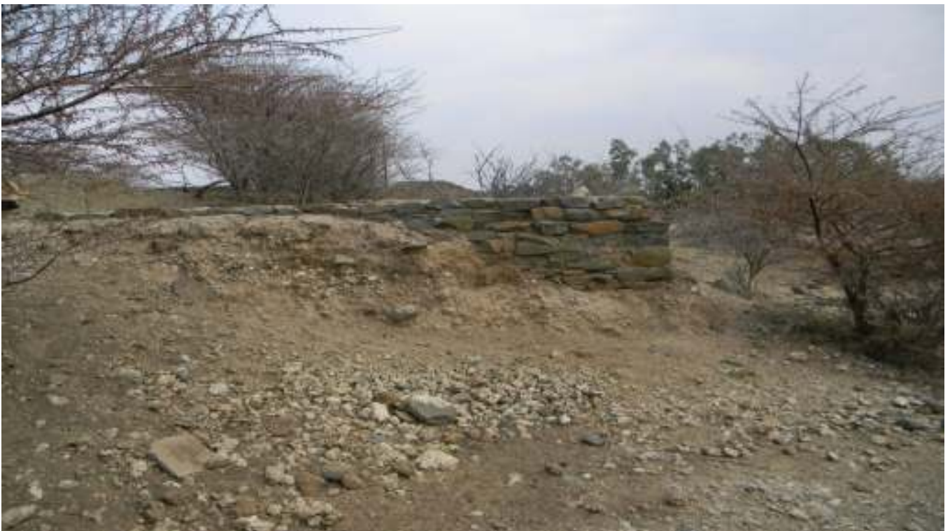
Figure 9: View of foundation of the derelict farm structure
