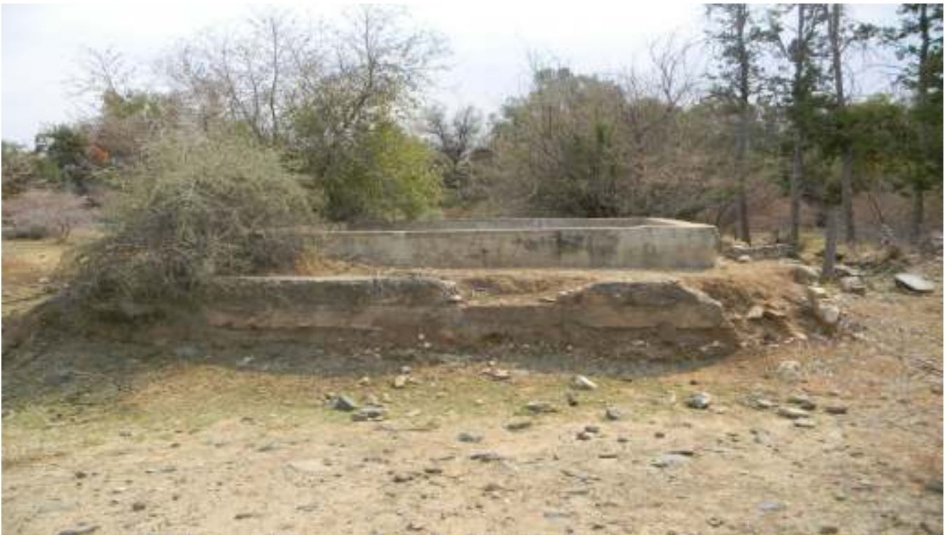
Figure 19: View of abandoned farm structure
