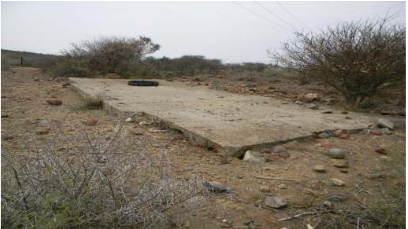
Figure 22: View of house floor of abandoned farm structure
