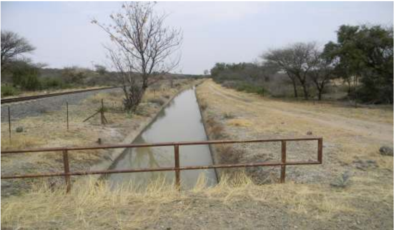
Figure 18: View of a canal cutting across the proposed prospecting site
